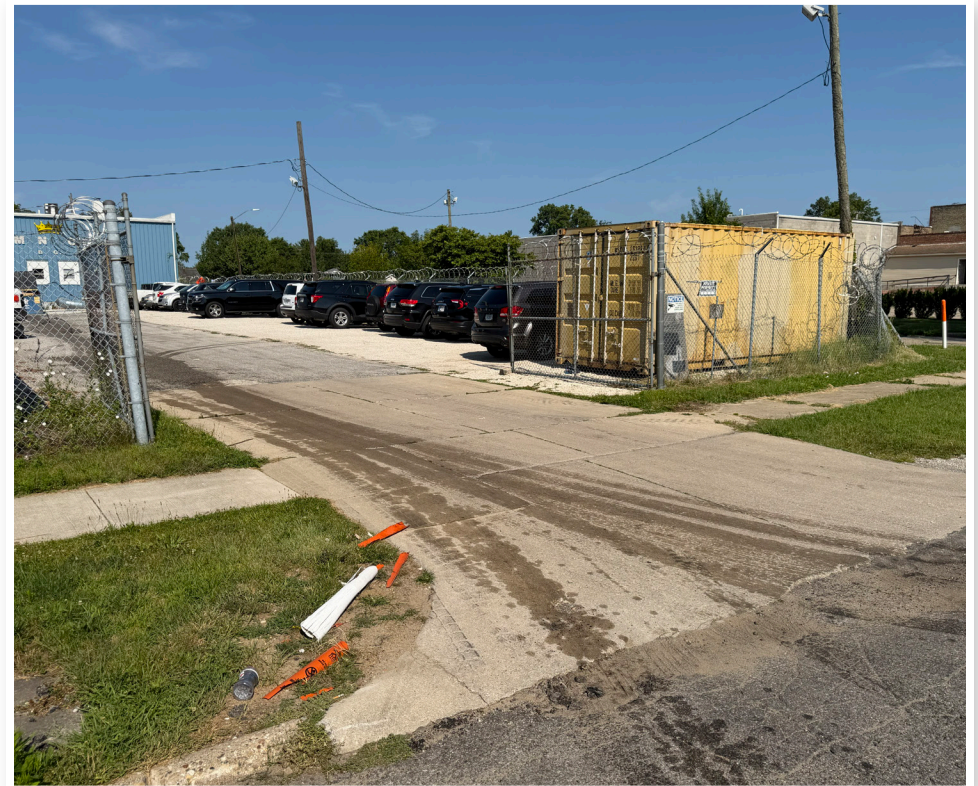
Business Entrance South of Rupel Intersection - Looking NW
