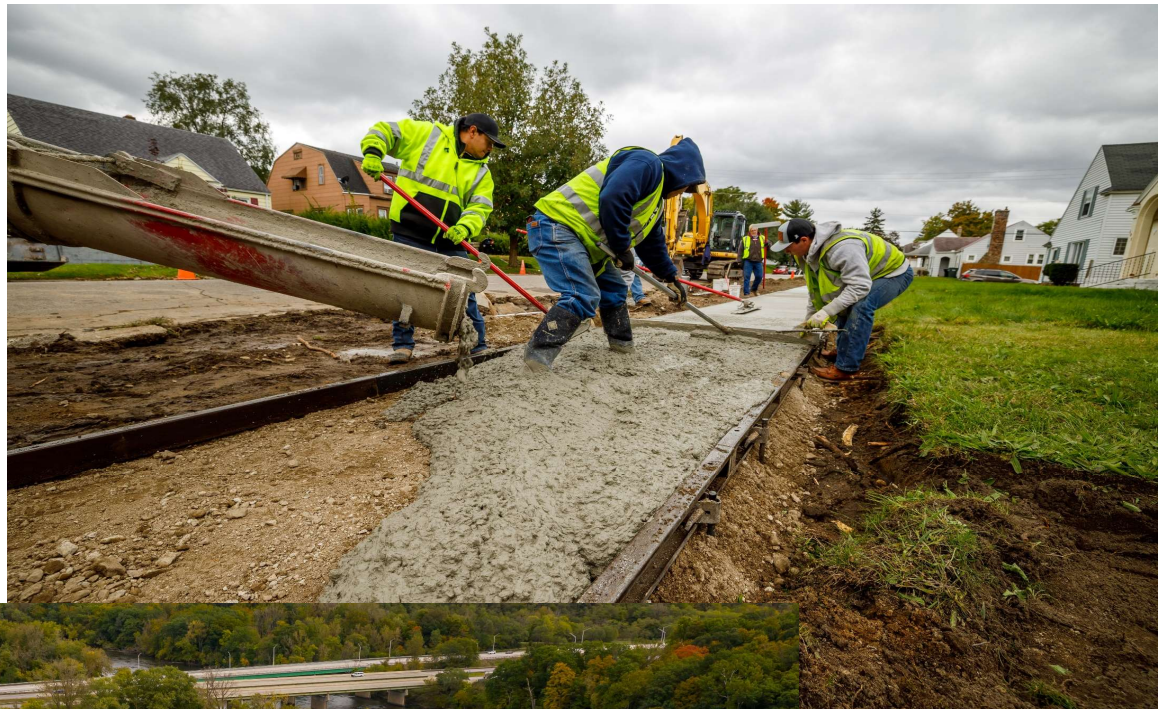
Curb & Sidewalk Program
