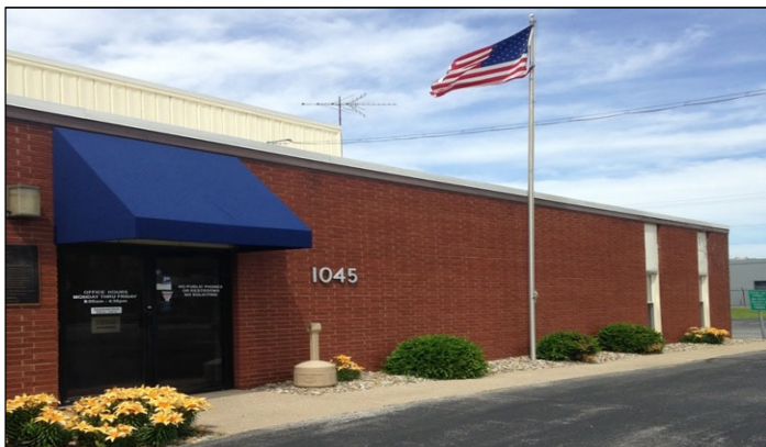
Central Services main office located at 1045 W Sample St
