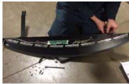
Light Bar Installation
