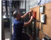
Working on Special Circuits
