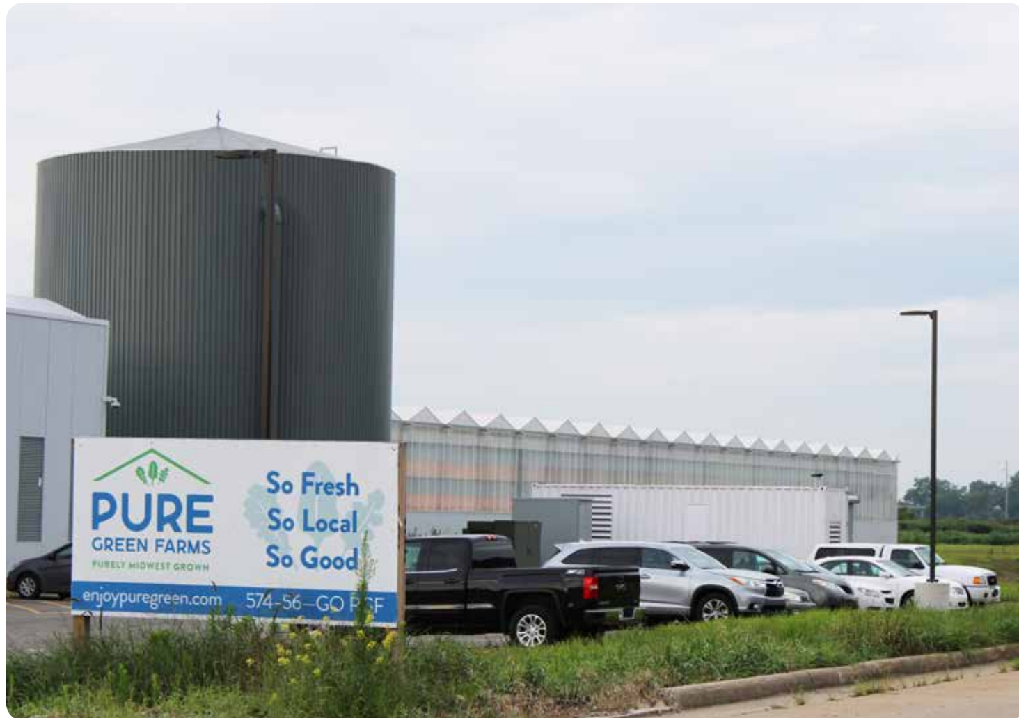
Pure Green greenhouse building.
