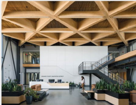
Hybrid Mass Timber/Structural Steel
