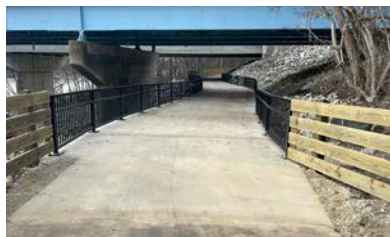
SAGAMORE PARKWAY TRAIL CONSTRUCTION INSPECTION WEST LAFAYETTE, INDIANA
