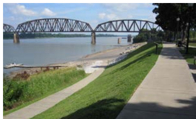
RIVERFRONT IMPROVEMENT PROJECTS HENDERSON, KENTUCKY
