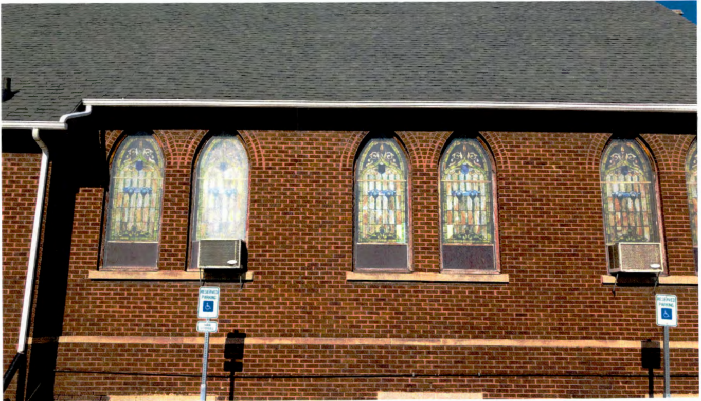
IMAGERY — East facade.
