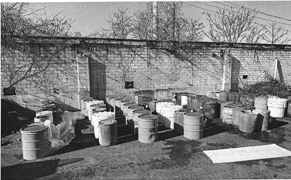
Photo 5: Drums stabilized and ready for sampling and disposal
