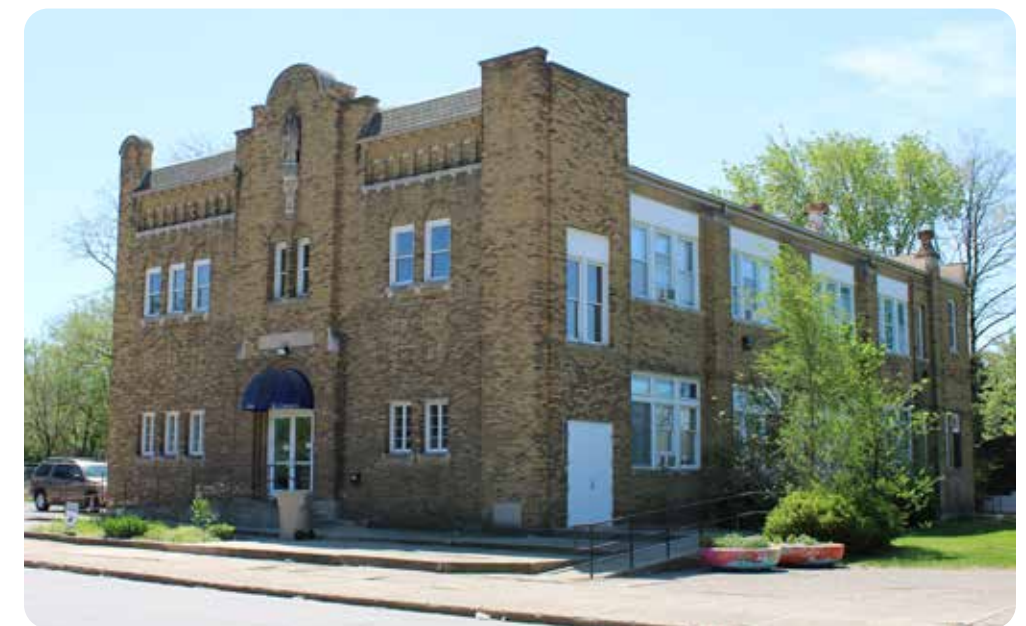
El Campito building.
