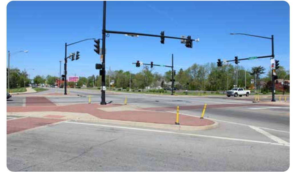
Western Avenue - Chapin Street intersection, looking northwest.
