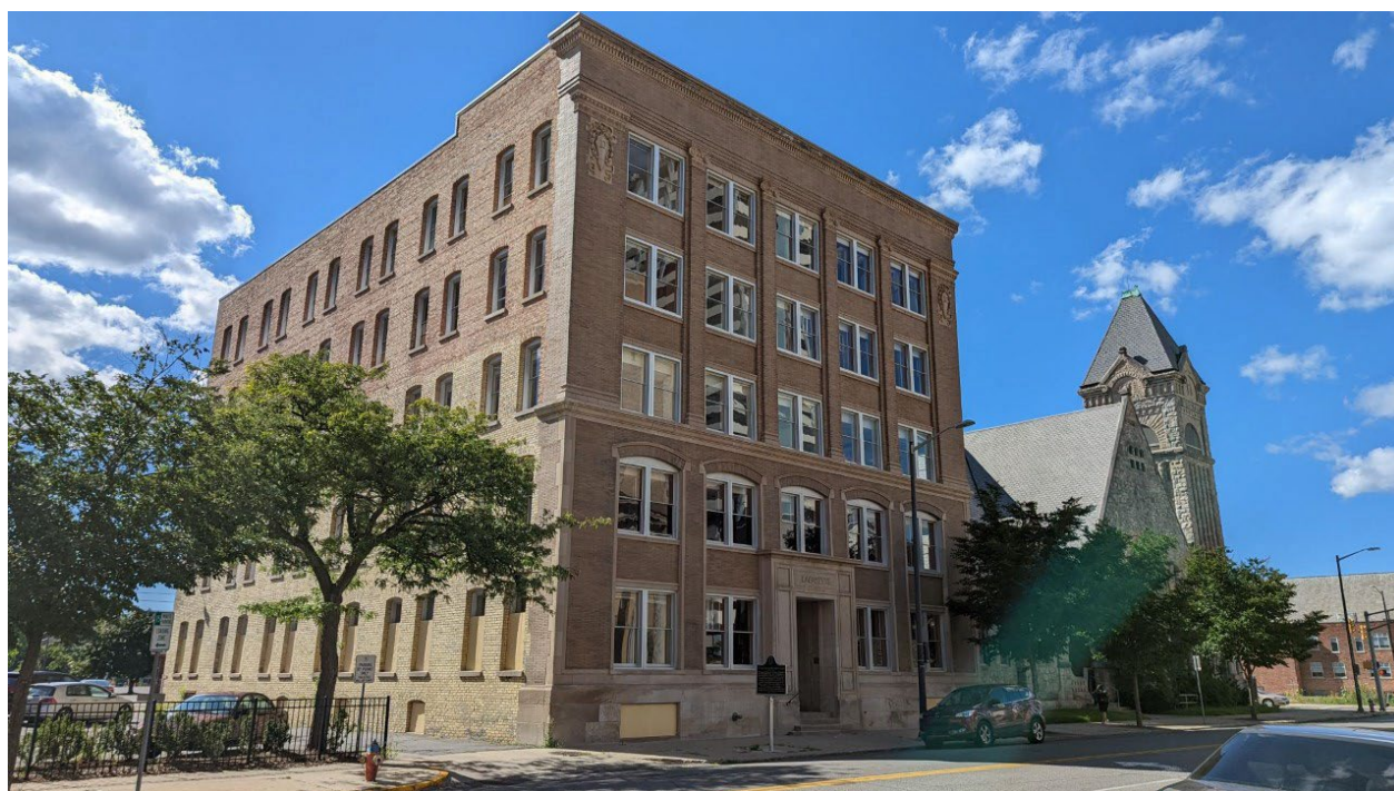
Figure 2. The Lafayette Building's east and south facing facades
