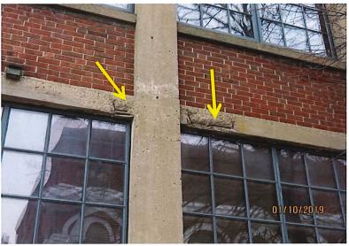
The vibrations from the adjacent construction had the potential to dislodge some of the loose concrete. It did not appear, however, that significant structural damage to the building could be attributed to this vibration. We would attribute the interior drywall cracks to the vibrations.
