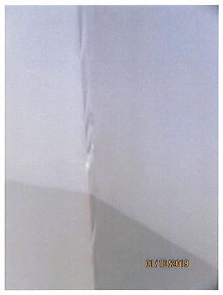
Also buckling could be seen in the upper corner of a drywall panel at the intersection with a concrete frame. It is highly likely the vibrations such as the occupants have described could cause this damage
