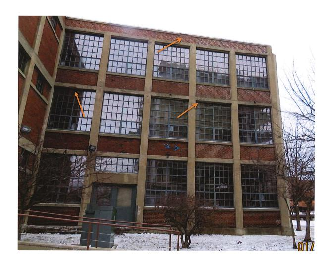
This is the chip at the top of the wall and a column with spalled concrete.
