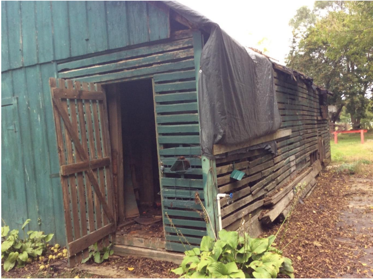
Figure 6 - Southwest corner of the corn crib.
