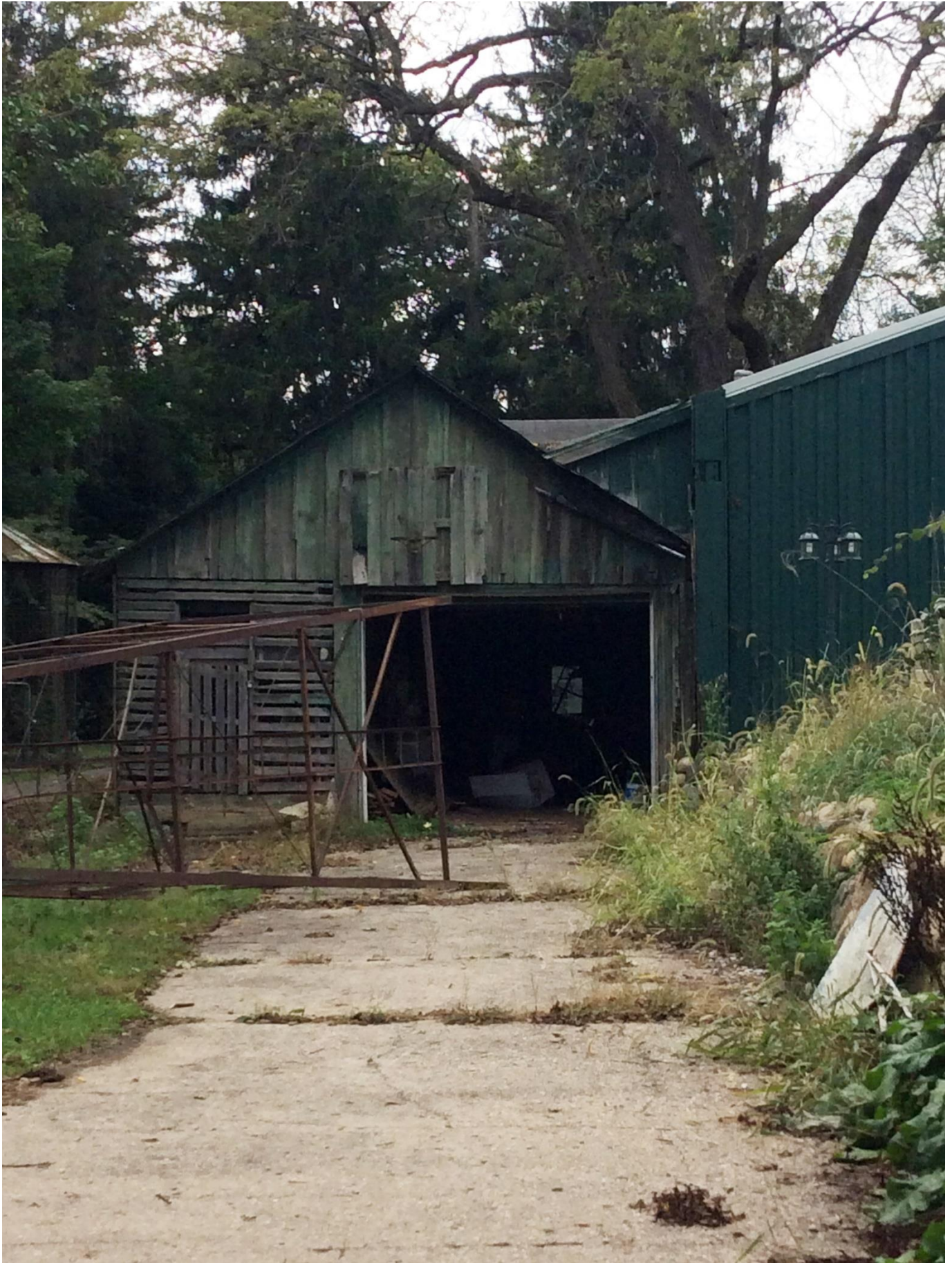
Figure 5 - Corn crib, east facade. Note roof eave.
