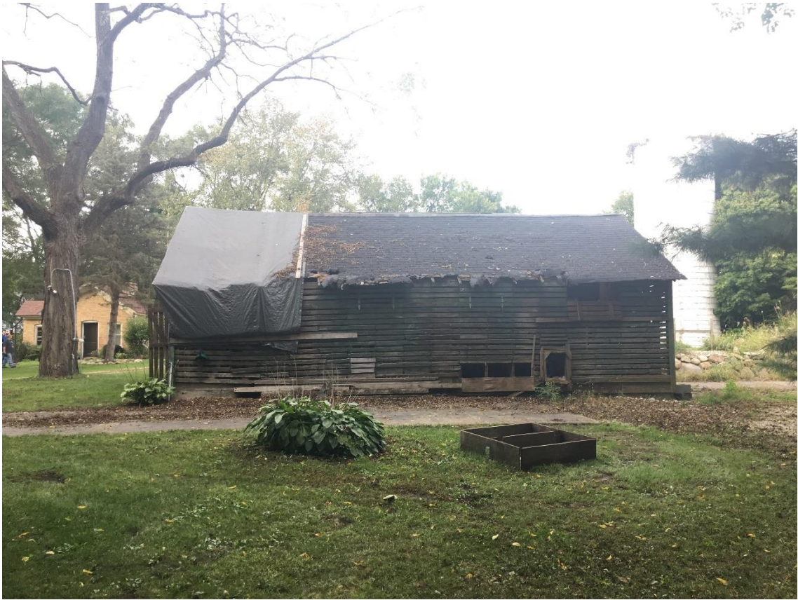
Figure 3 - Corn crib, south facade.
