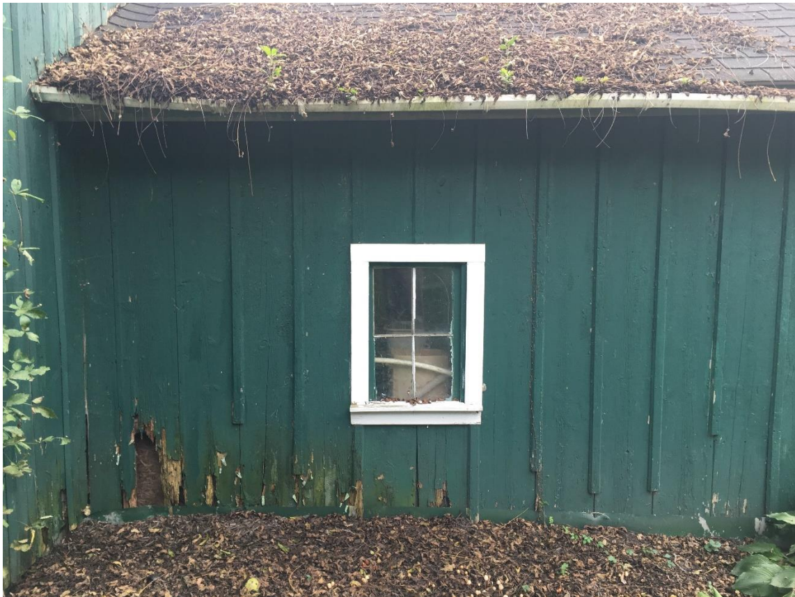
Figure 4 - Corn crib, north facade.
