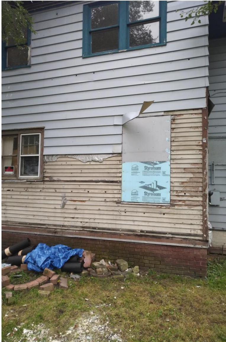
Figure 6 – 760 Portage, side. Aluminum siding removal.
