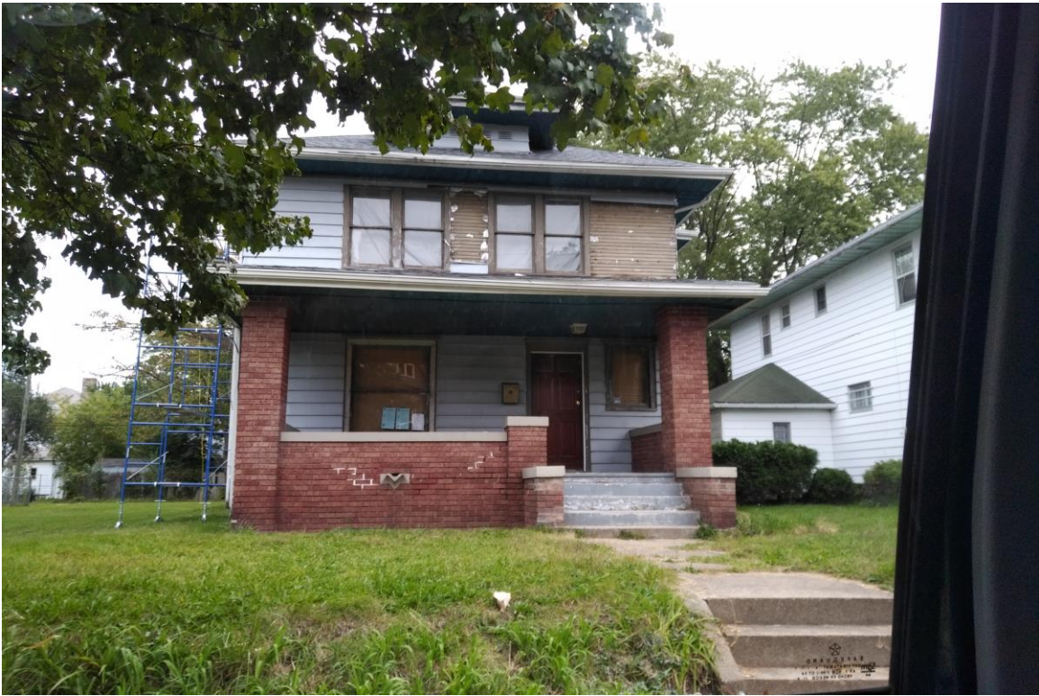
Figure 4 – 760 Portage, front. Aluminum siding removal.
