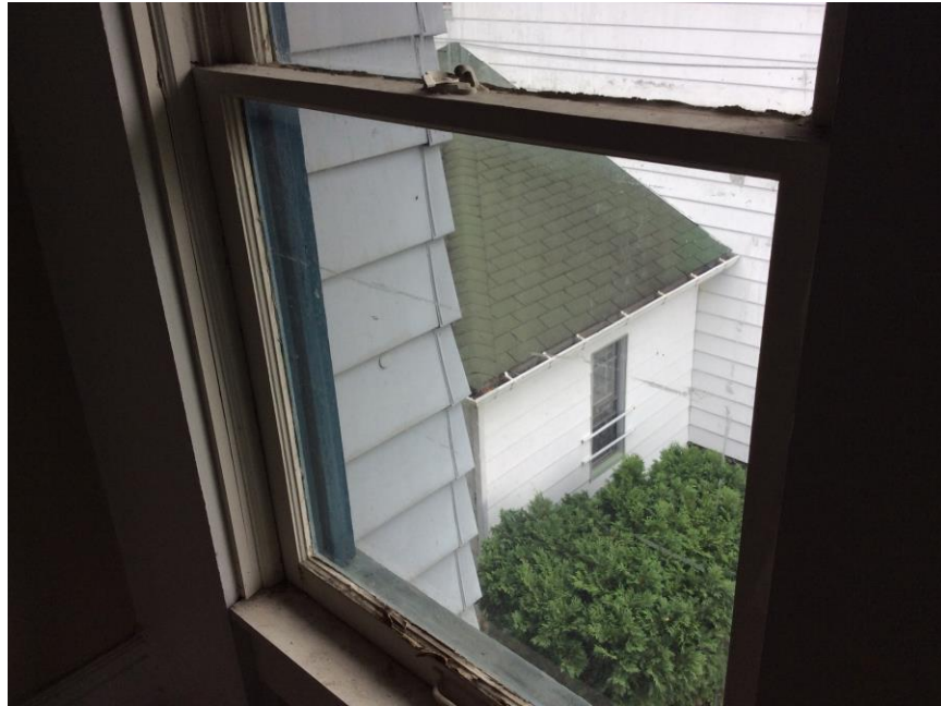
Figure 7 – 760 Portage. Existing window.
