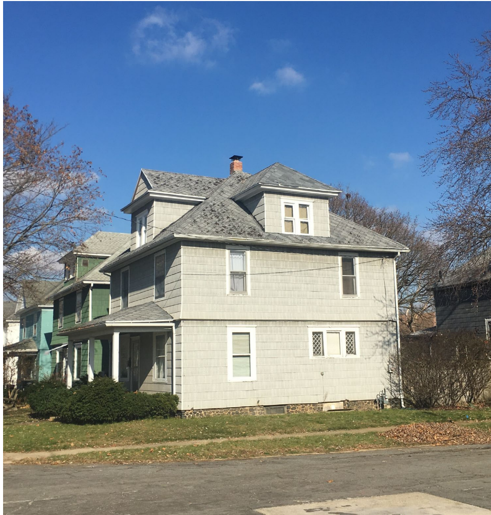
Figure 2 - 702 N St Joseph, looking north, northeast.
