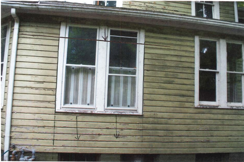
Figure 4—720 Park, kitchen windows
