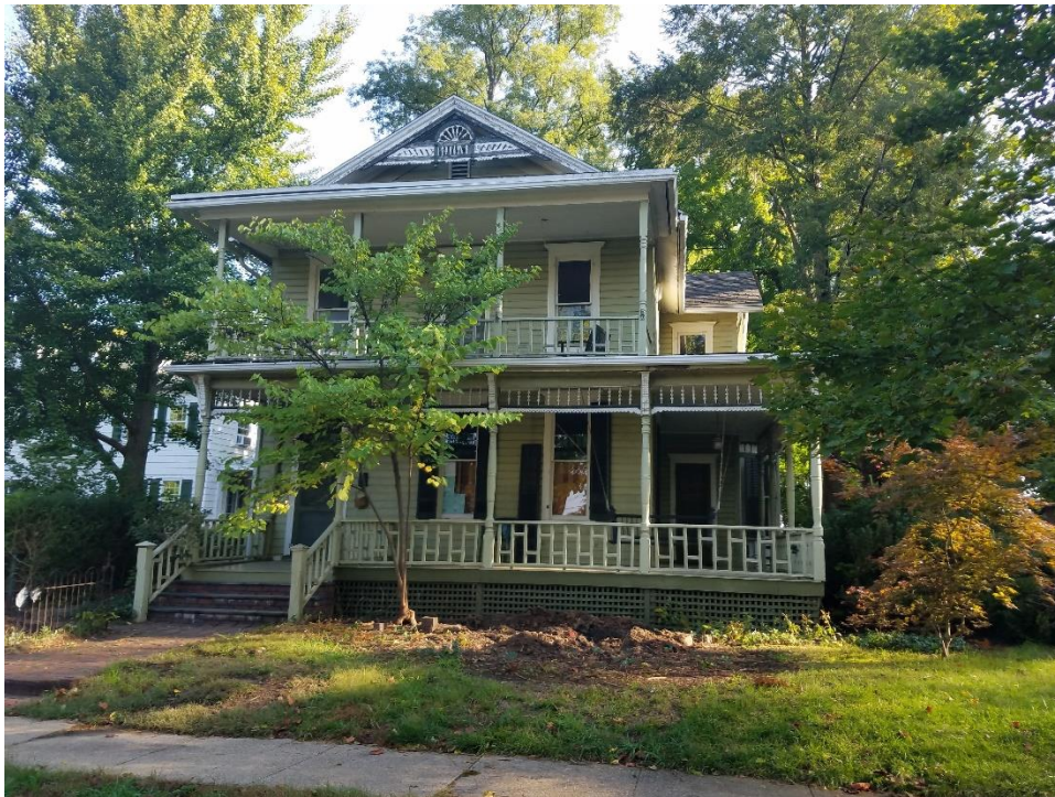
Figure 1—720 Park, looking north east
