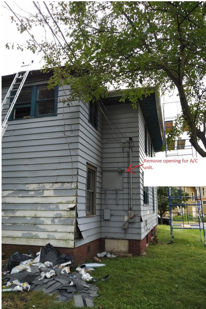
Figure 2 – 760 Portage, looking south west. Window proposed for removal is visible at center.
