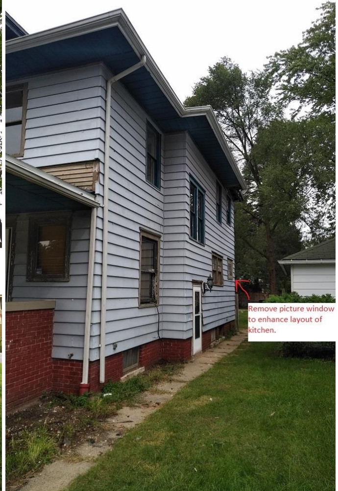
Figure 3 – 760 Portage, looking north. Window proposed for removal is visible at left.
