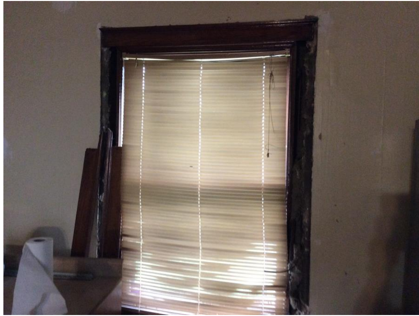
Figure 9 – 760 Portage. Existing window.
