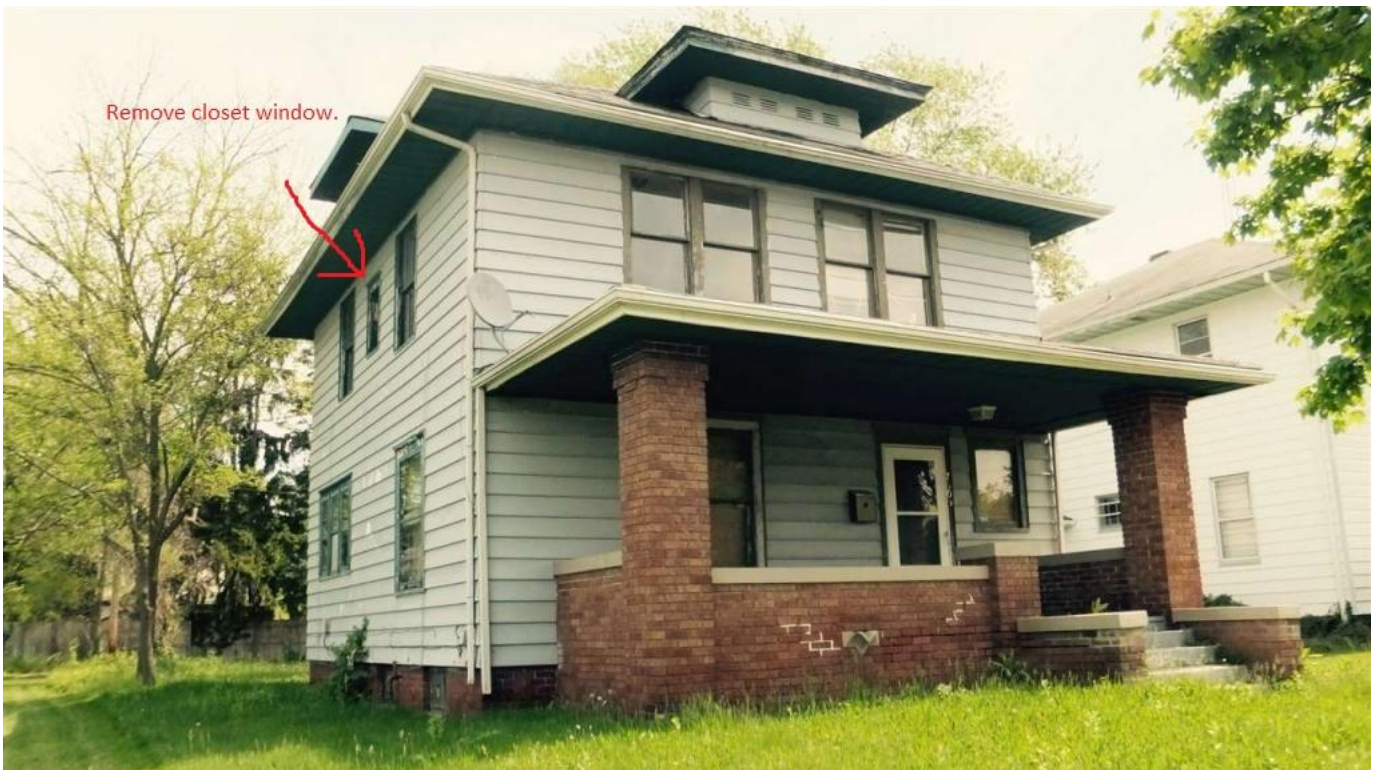
Figure 1 – 760 Portage, from sidewalk, looking north east. Window proposed for removal is visible at left.
