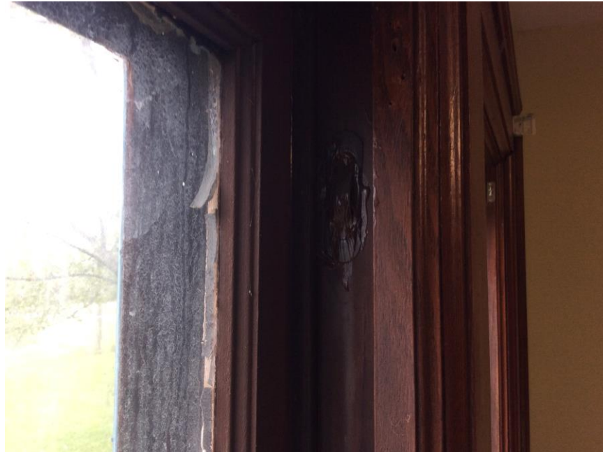
Figure 8 – 760 Portage. Existing window.
