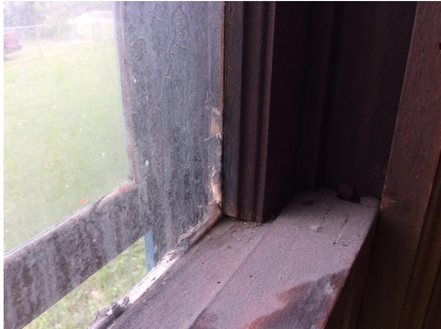
Figure 10 – 760 Portage. Existing window.
