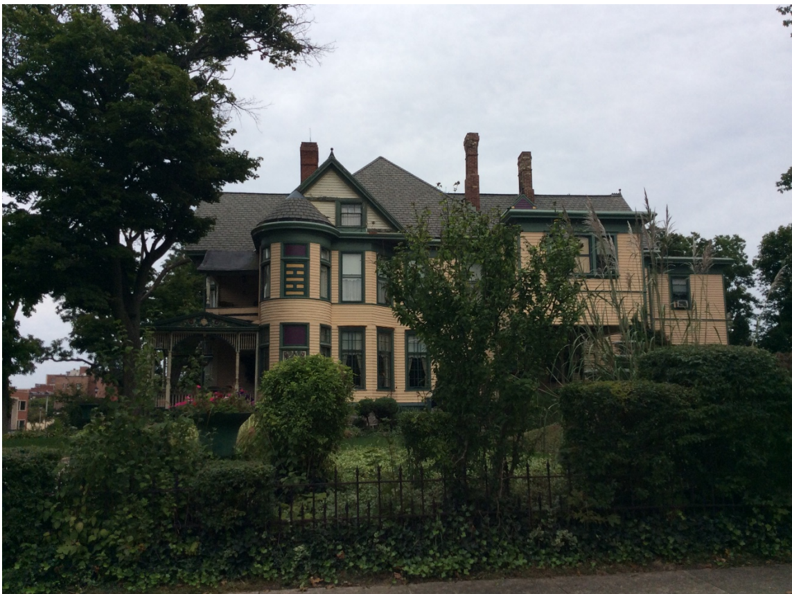
Figure 2 – 630 W Washington the sidewalk on Scott Street, looking east..
