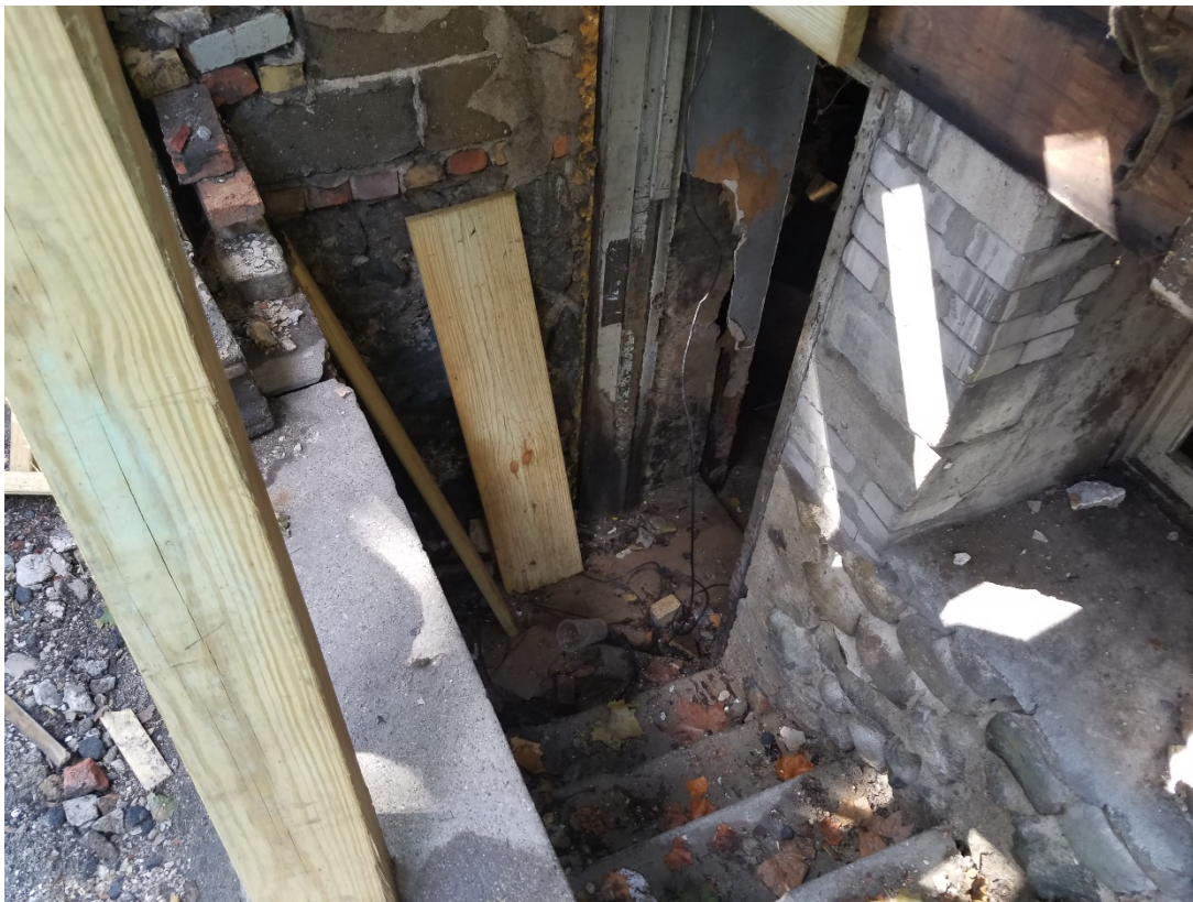
Figure 5 - Basement access beneath stairwell.
