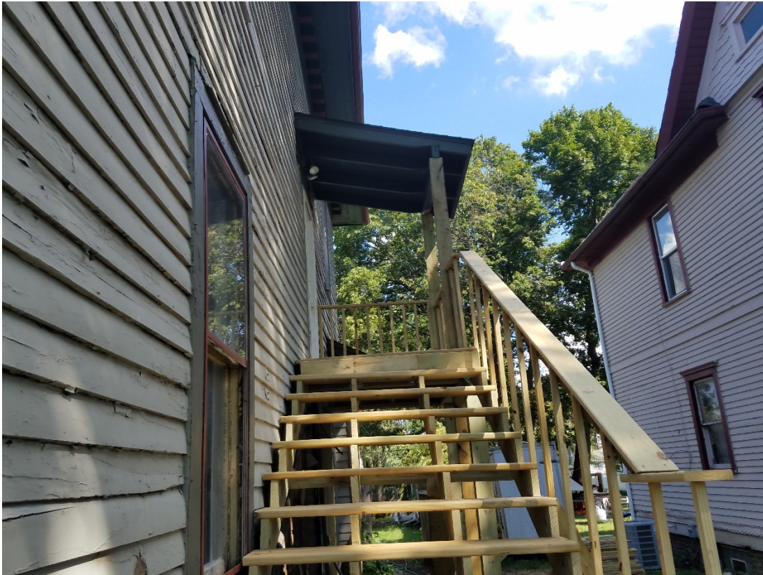
Figure 4 - Rebuilt stairwell, looking east.
