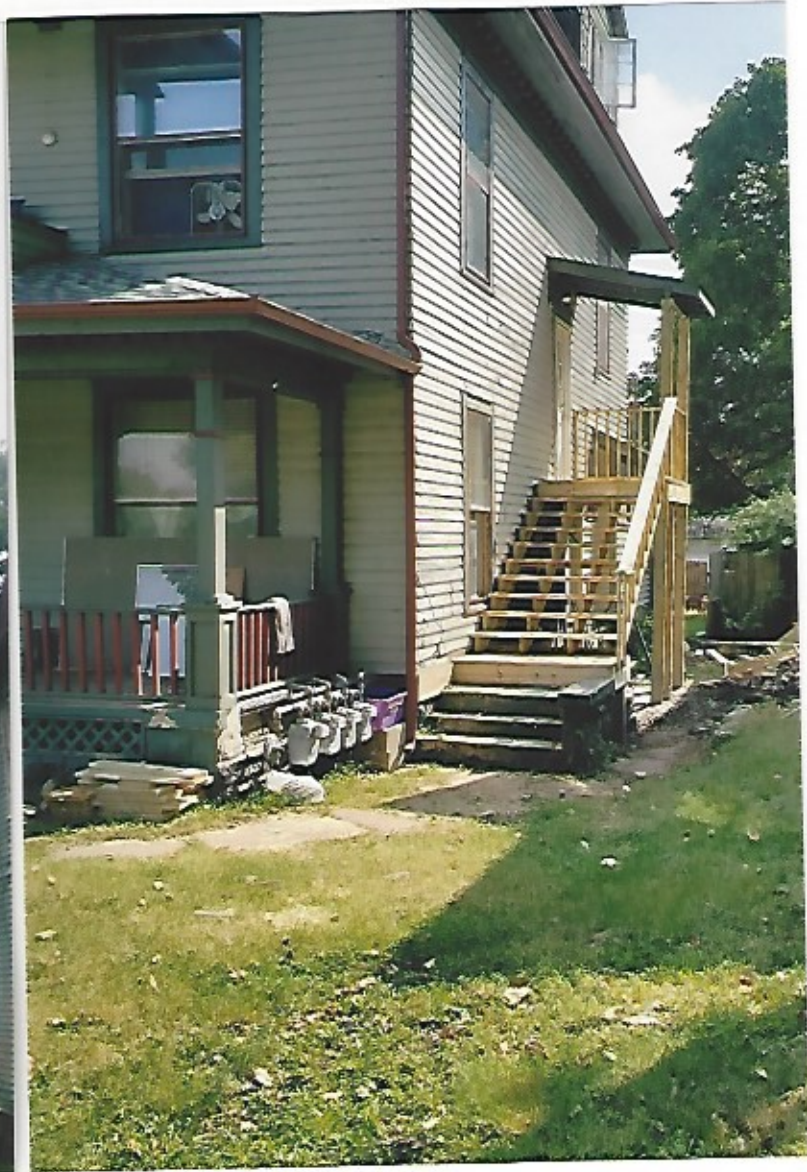
NEW REPAIRED STEPS
