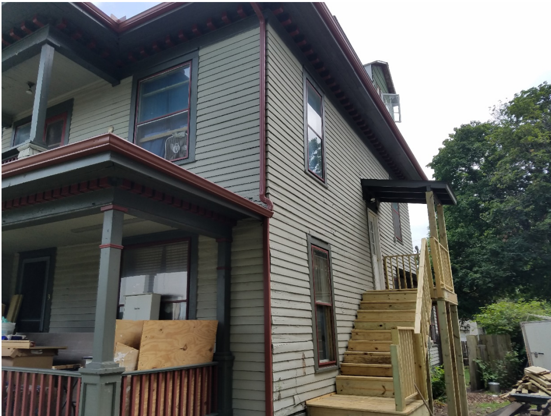
Figure 3 - Close-up of the stairs.
