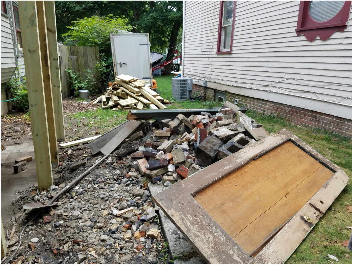
Figure 6 - Deconstructed stone and brick wall.
