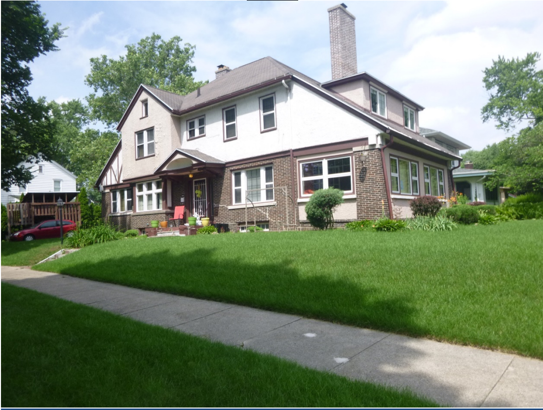
Figure 1-- 815 Arch Avenue, looking west towards the main house from near the intersection of Arch Avenue and Riverside Drive.
