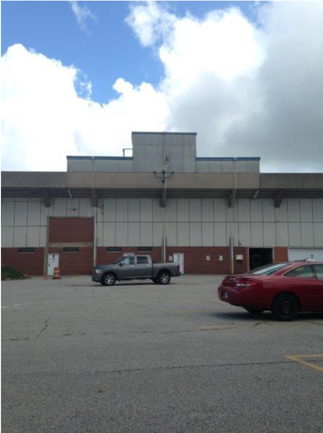
Figure 5 - Rear of the press box, where application item 1) will be installed.
