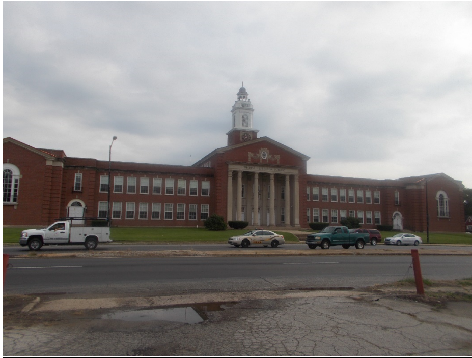
Figure 1- The Thomas Jefferson School main building stands to the south of the application area, seen from a Staff photograph. All remaining photos courtesy of the applicant.
