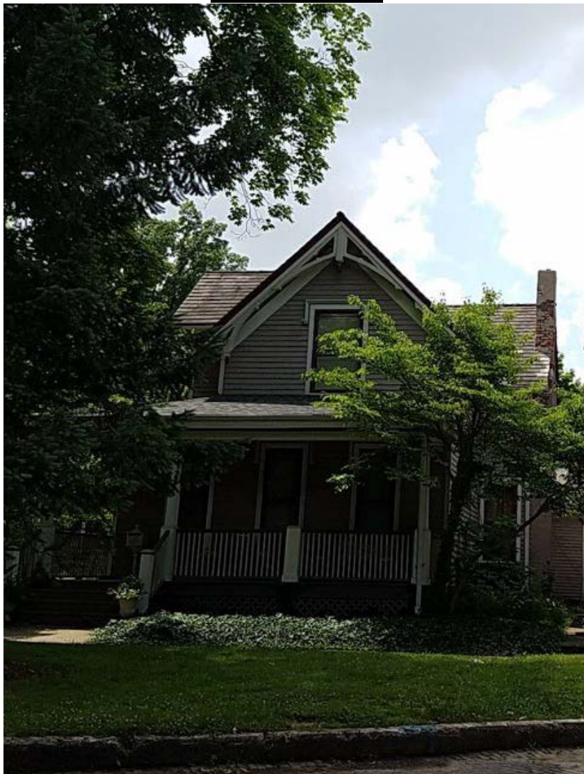
Figure 1 -- 801 Park from the street, looking west. The subject chimney is visible along at right.
