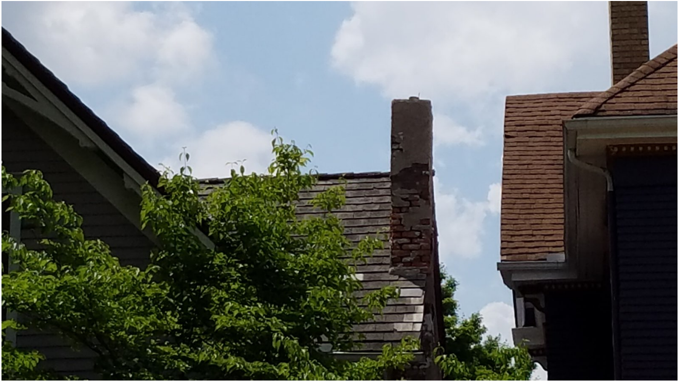
Figure 2 -- Close-up of the chimney at the northeast corner of the structure.
