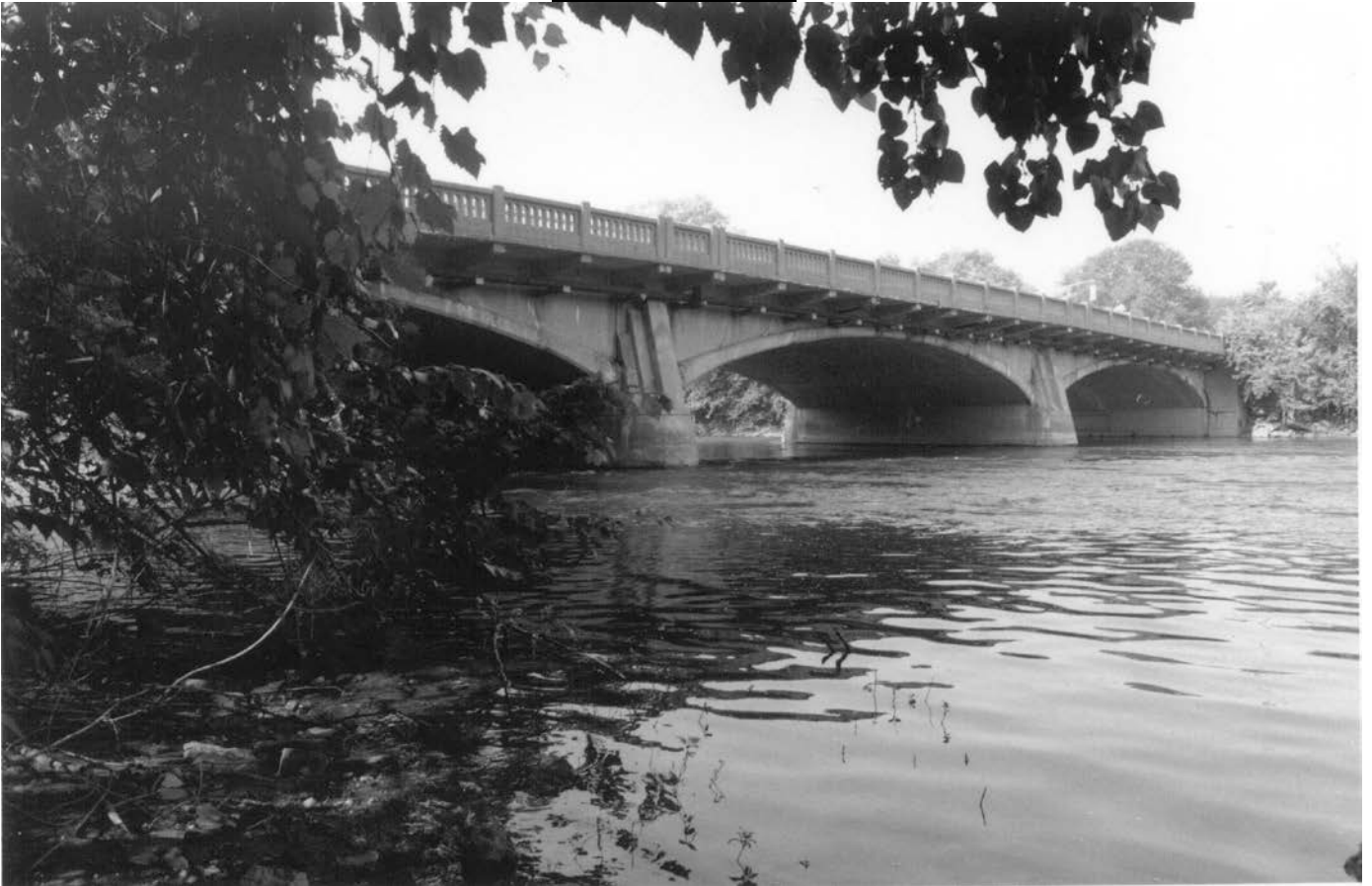
Figure 1 - Angela Boulevard Bridge, looking southwest.
