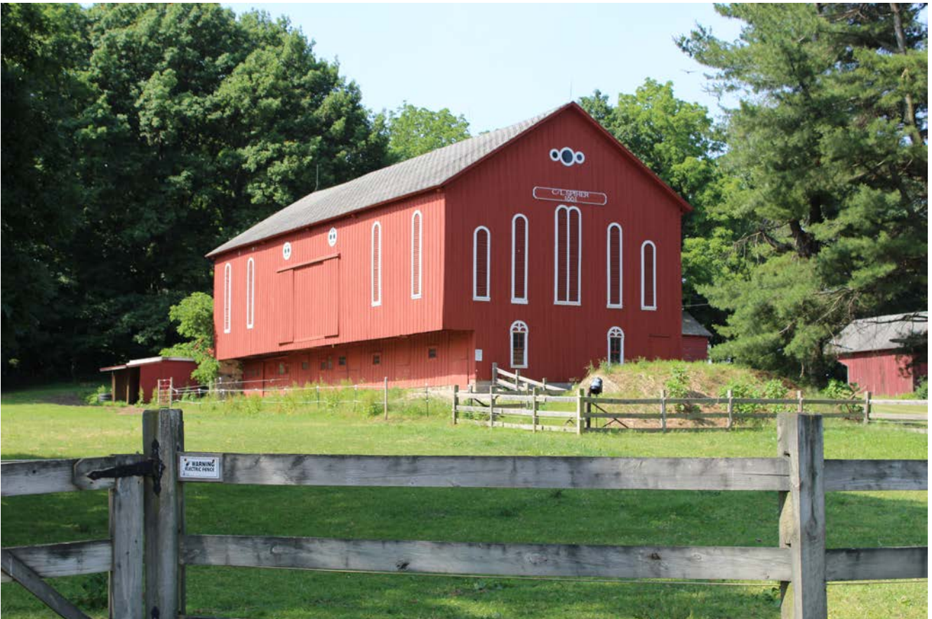
Figure 2 - The 1880 barn, looking south-southwest from Old Cleveland Road.
