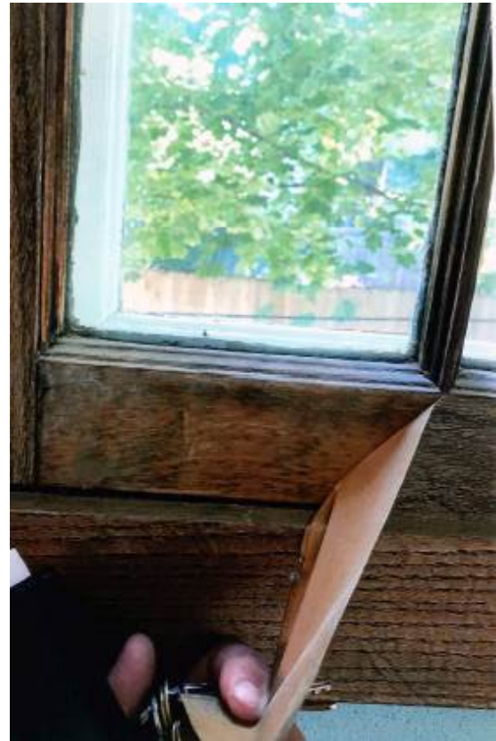
Figure 8 – Peeling veneer
