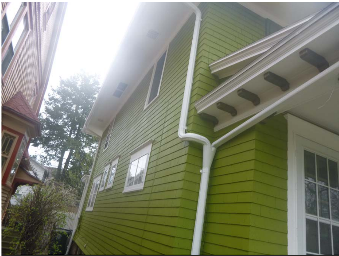
Figure 2 - 608 Park, north face. Window #1, #2, #3, and #4 are visible.
