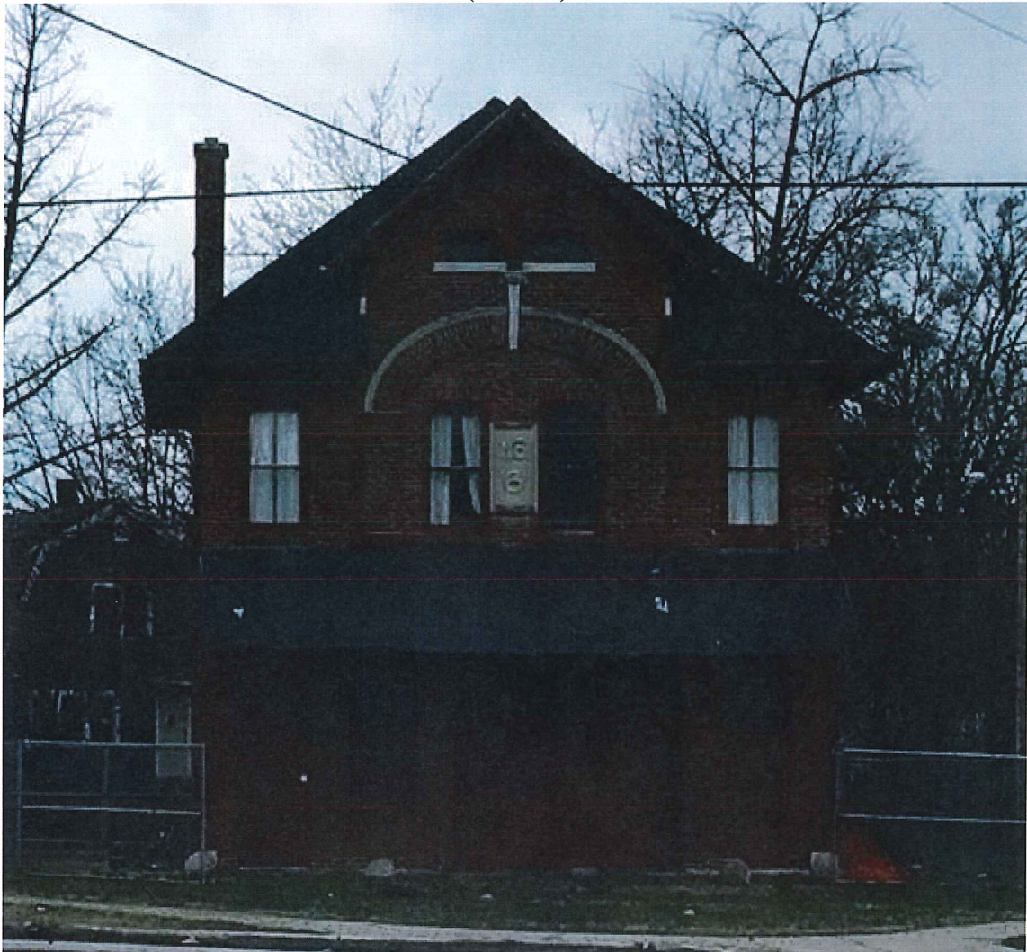
EAST (FRONT) VIEW
