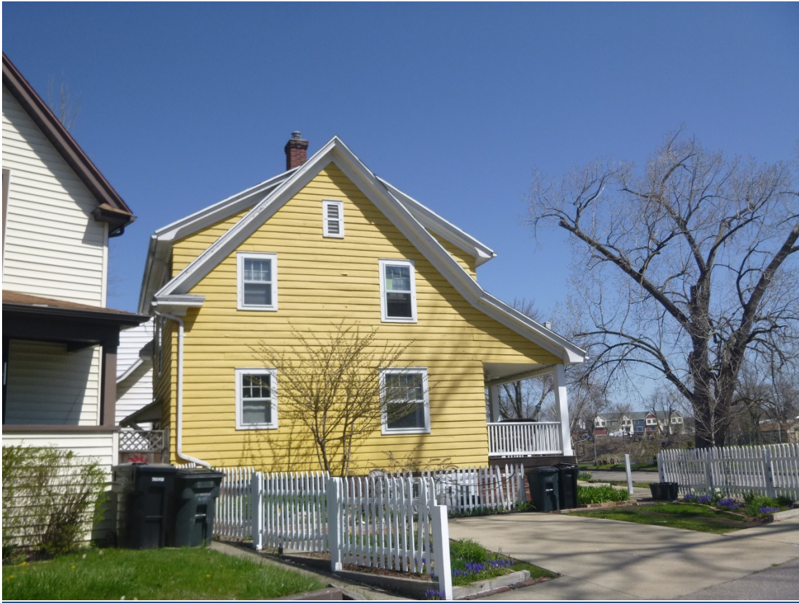
Figure 3 - South face of 619 Edgewater, April 30, 2018
