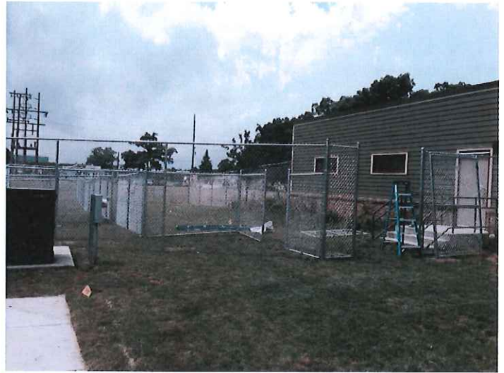
Play Yard during construction.
