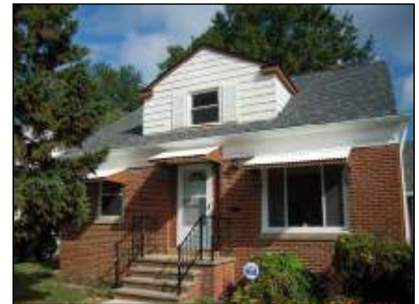
fig. 48 CCLRC has this property for sale after rehabilitation
