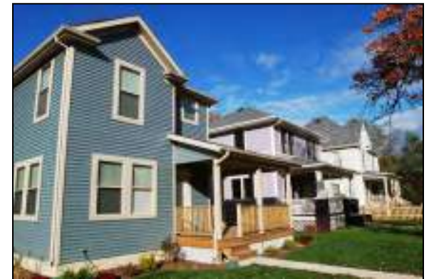
fig. 57 A newly constructed Habitat home
