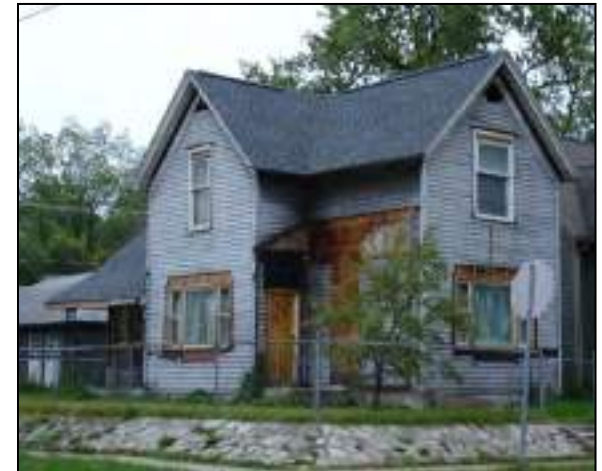
fig. 44 Dilapidated vacant homes have a negative impact on a neighborhood (before)
