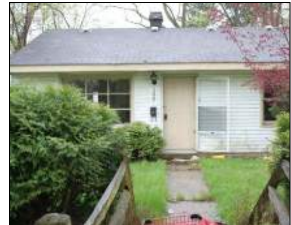
fig. 25 Not all properties are easily categorized as demolition vs. repair candidates by looking at the exterior
