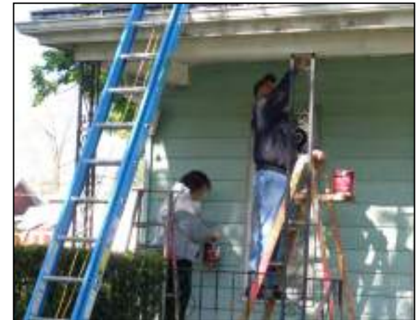
fig. 4 The community works to repair homes through Rebuilding Together
