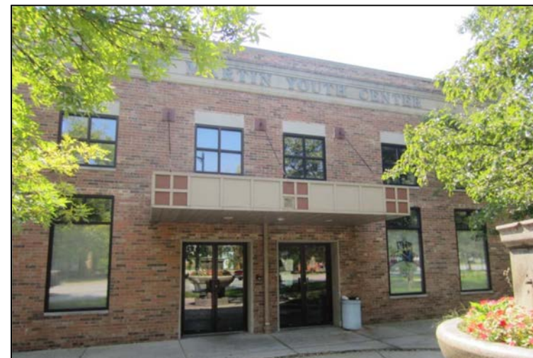
Photo 3 - As part of the Colfax Campus, the Charles Martin Center is a centerpiece for the neighborhood
