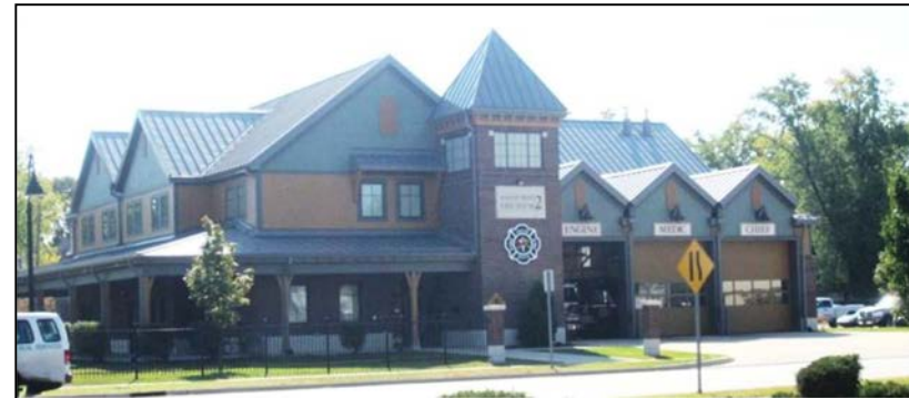
Photo 16 - Fire Station # 2 – The City of South Bend’s newest fire station and a strong neighborhood asset
