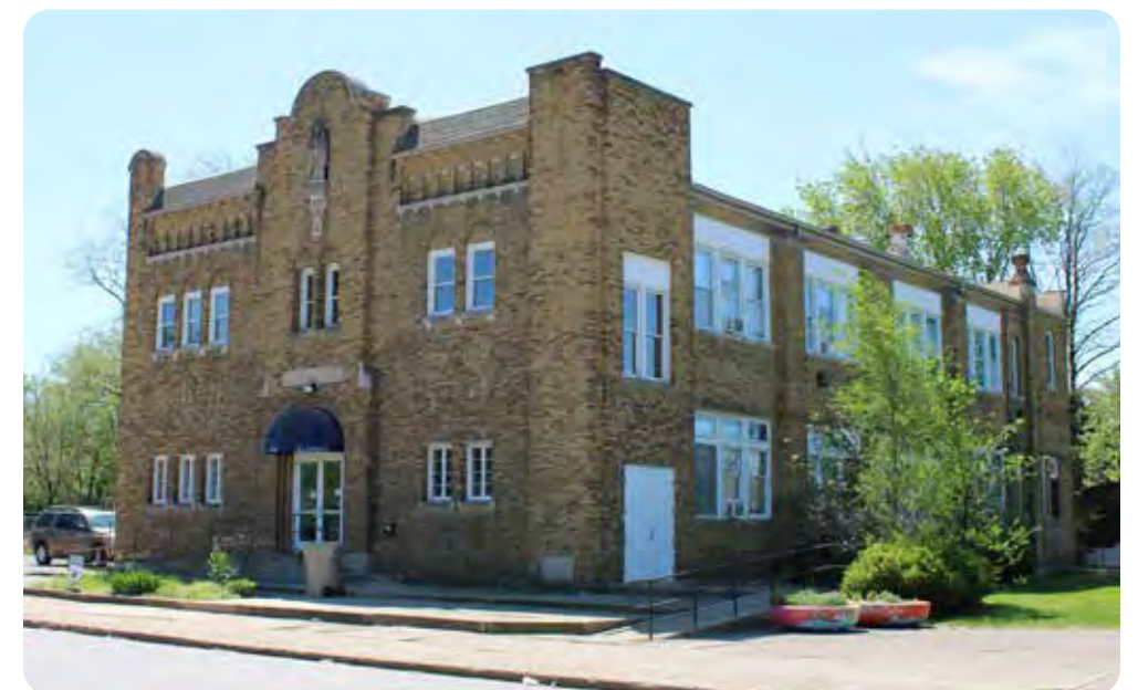
El Campito building.
