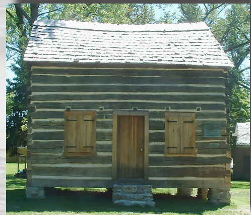
The cabin post restoration.
