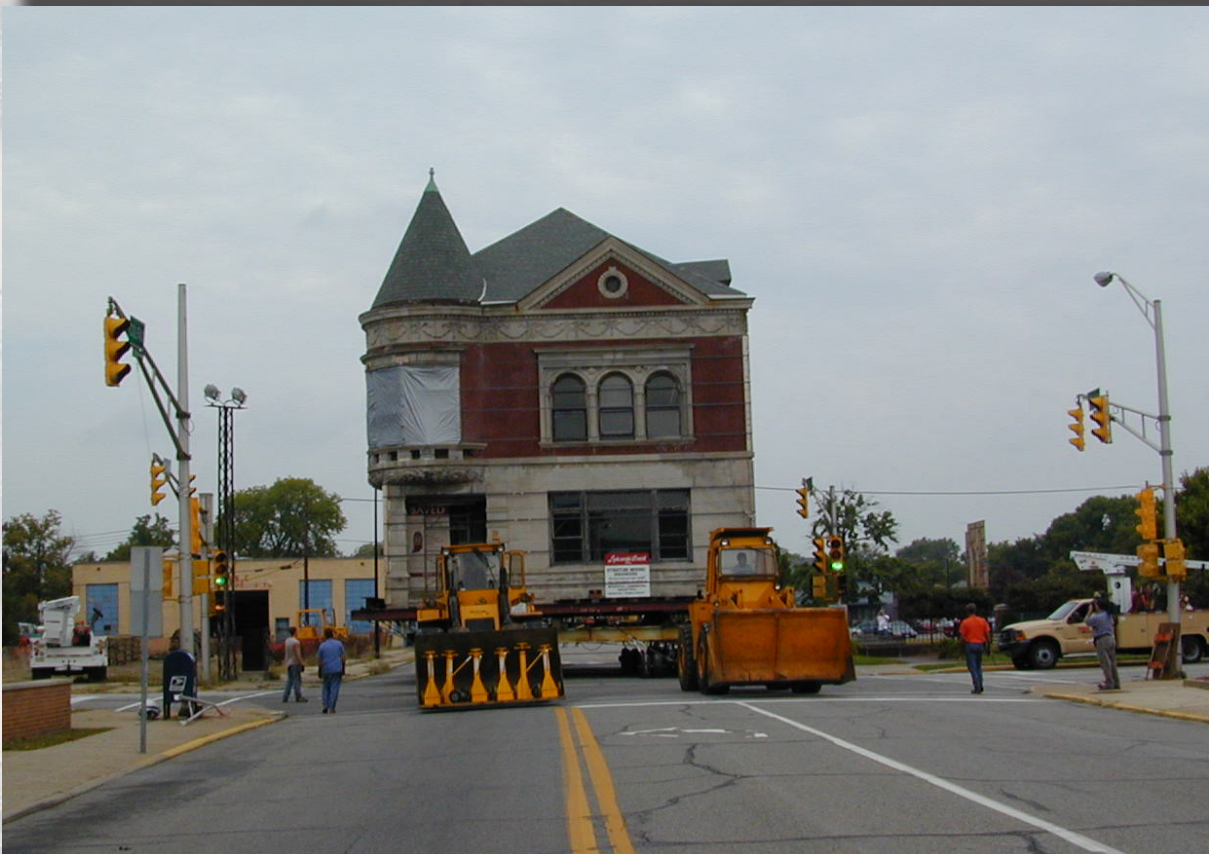
Lykowski Construction moving the Remy Building
