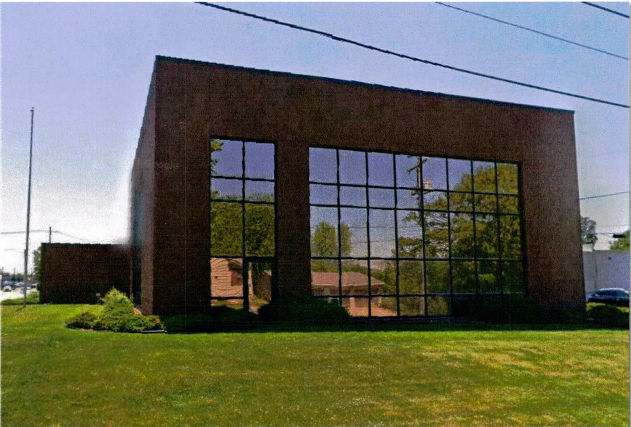
View of the Nexus Center looking south from Sherwood Street
