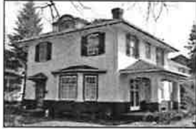
616 Park Avenue American Foursquare
