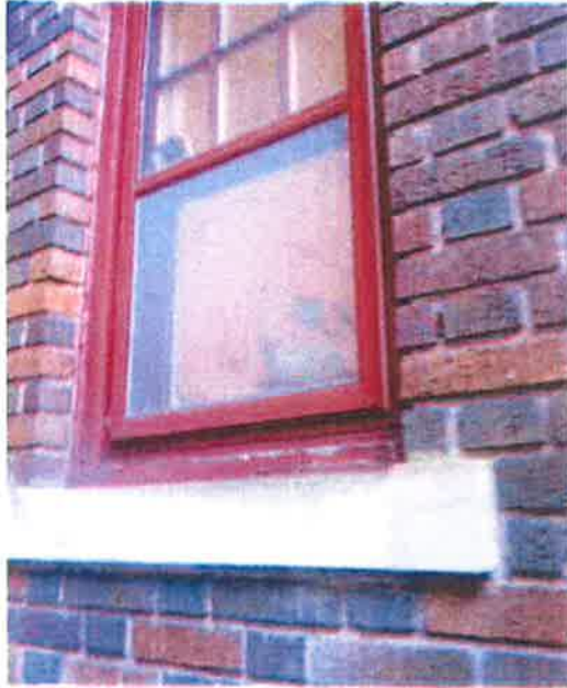
HOUSE - WINDOW CASING, SIDE C
