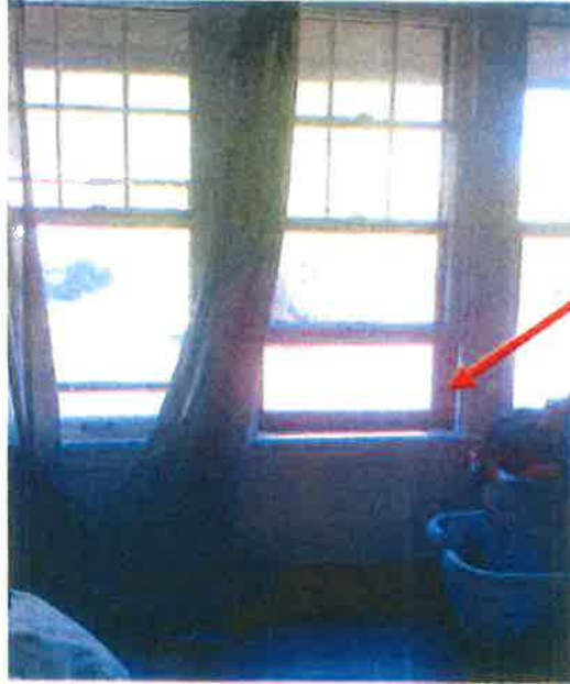
BEDROOM 5 - WINDOW JAMB, SIDE A
