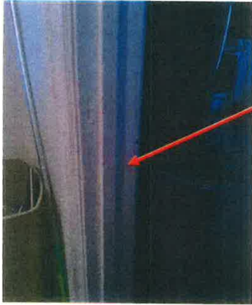
KITCHEN - DOOR CASING, SIDE D
