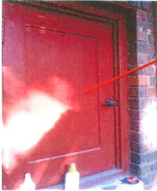
HOUSE - ELECTRIC BOX DOOR, SIDE C
