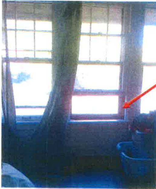
BEDROOM 5 - WINDOW JAMB, SIDE A
