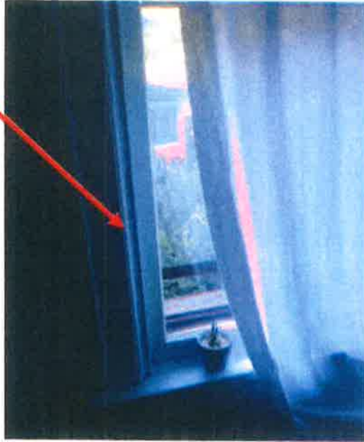
BEDROOM 2 - WINDOW CASING, SIDE A
