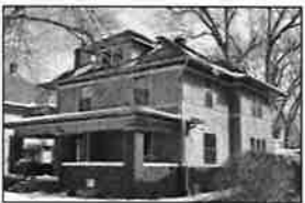
810 Leland Avenue American Foursquare/Prairie Style
