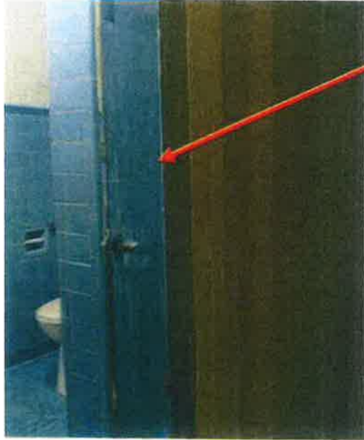
BATHROOM - DOOR JAMB, SIDE B
