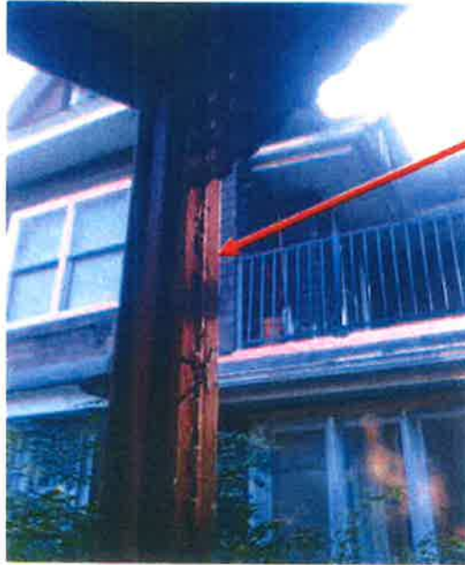
HOUSE - POST, SIDE C
