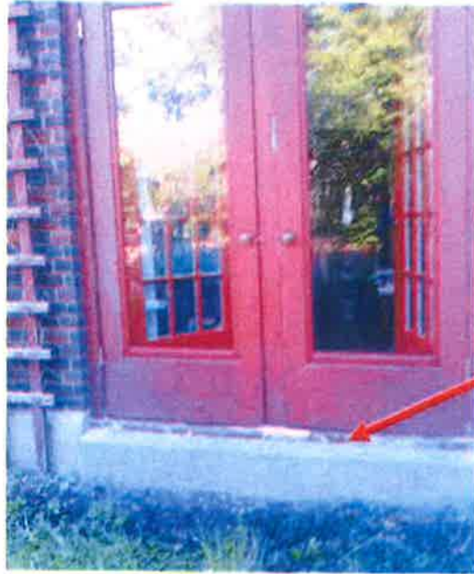
HOUSE - DOOR THRESHOLD, SIDE A
