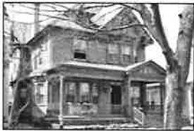
803 Park Avenue Queen Anne: Half-timbered
