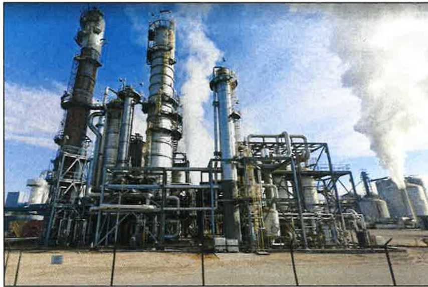
View Looking North from West Calvert Street
