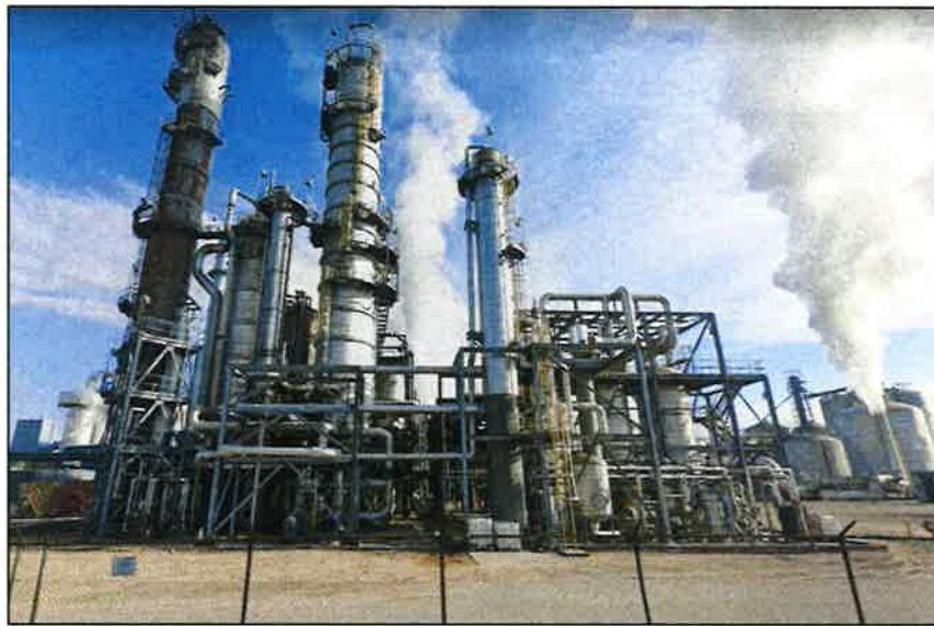
View Looking North from West Calvert Street
