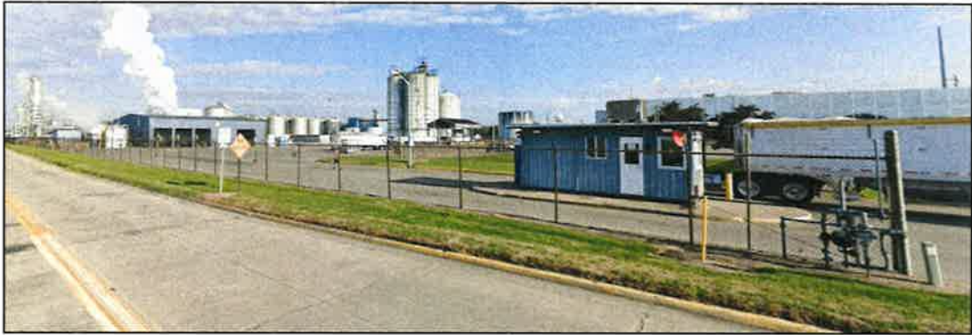
View Looking Northwest from West Calvert Street
