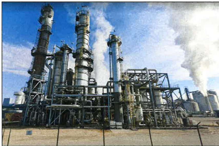
View Looking North from West Calvert Street
