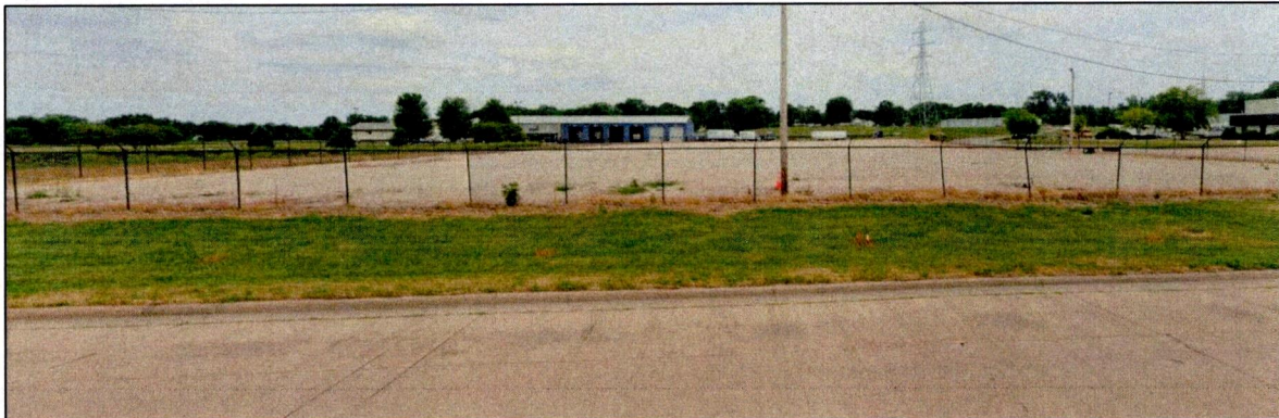
View of 3161 Youngs Court looking east from New Energy Drive
