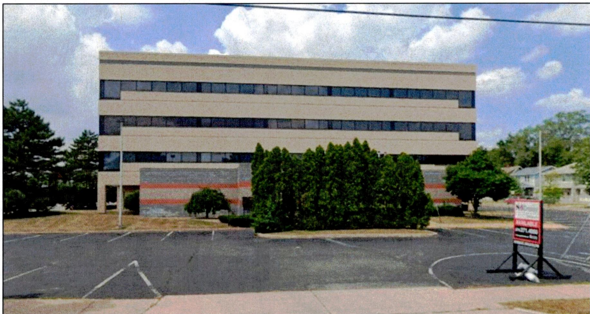
View from Notre Dame Avenue looking west
