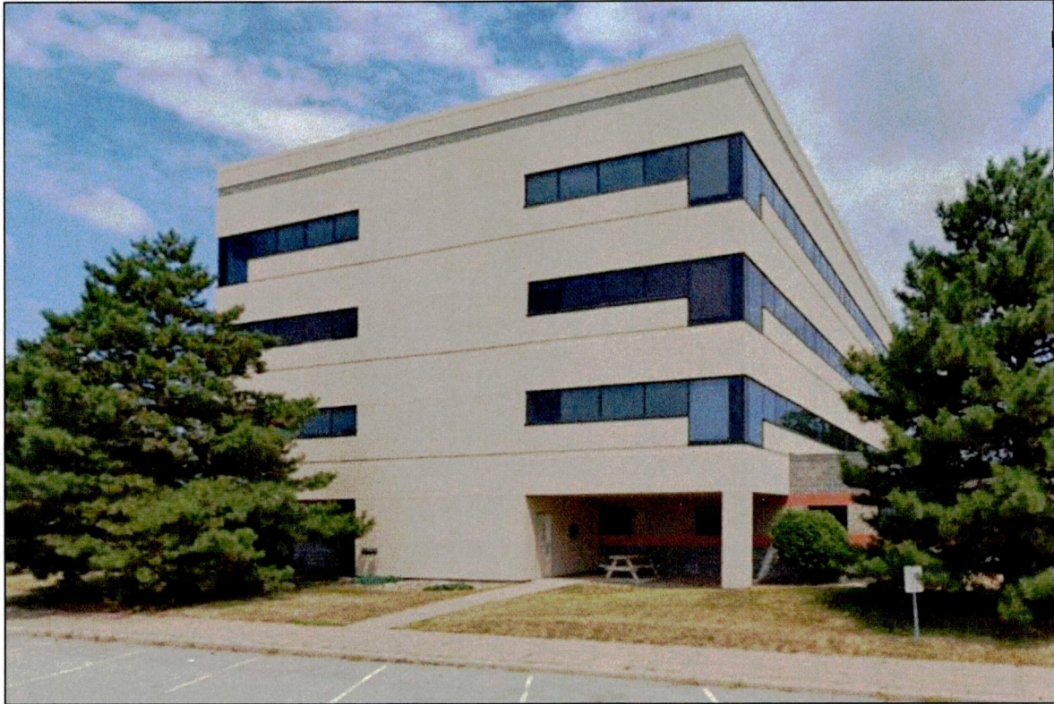
View from Cedar Street looking north
