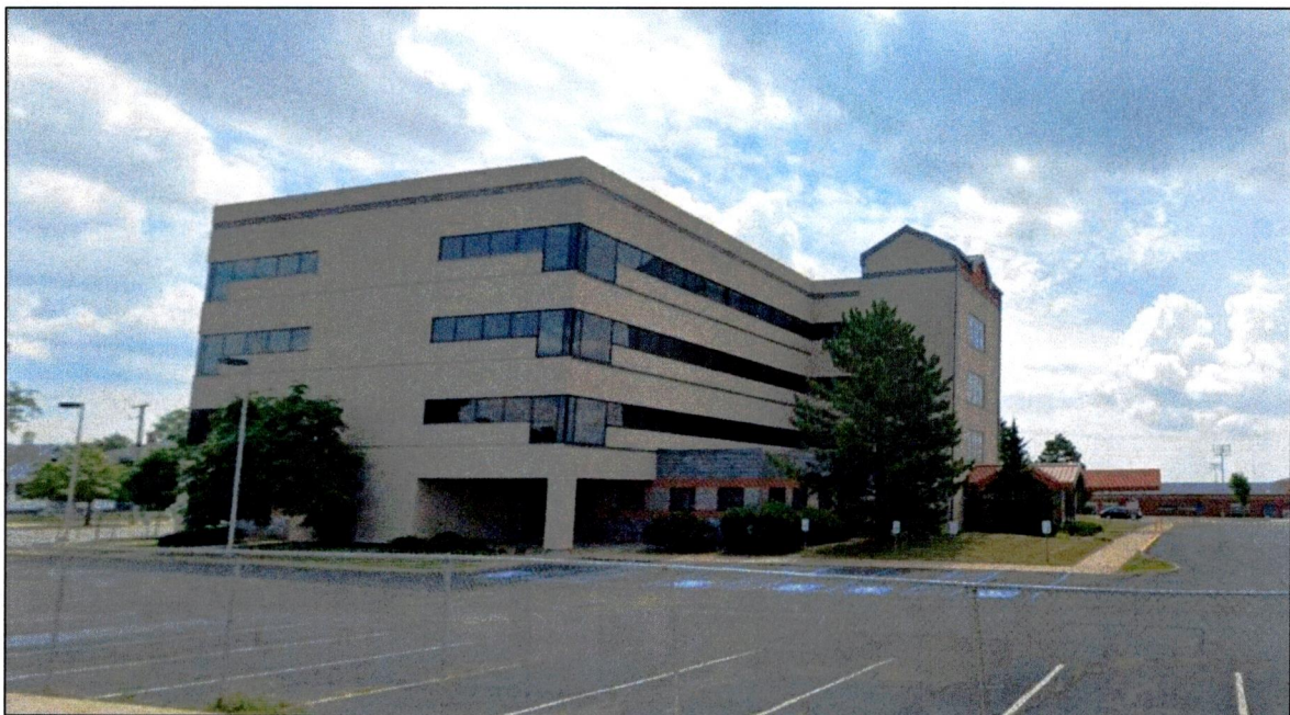
View from Miner Street looking south-southeast
