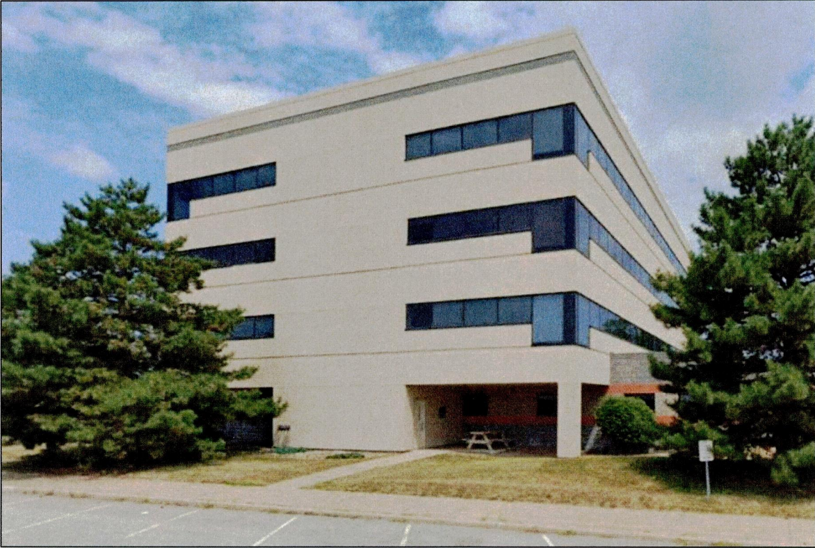
View from Cedar Street looking north
