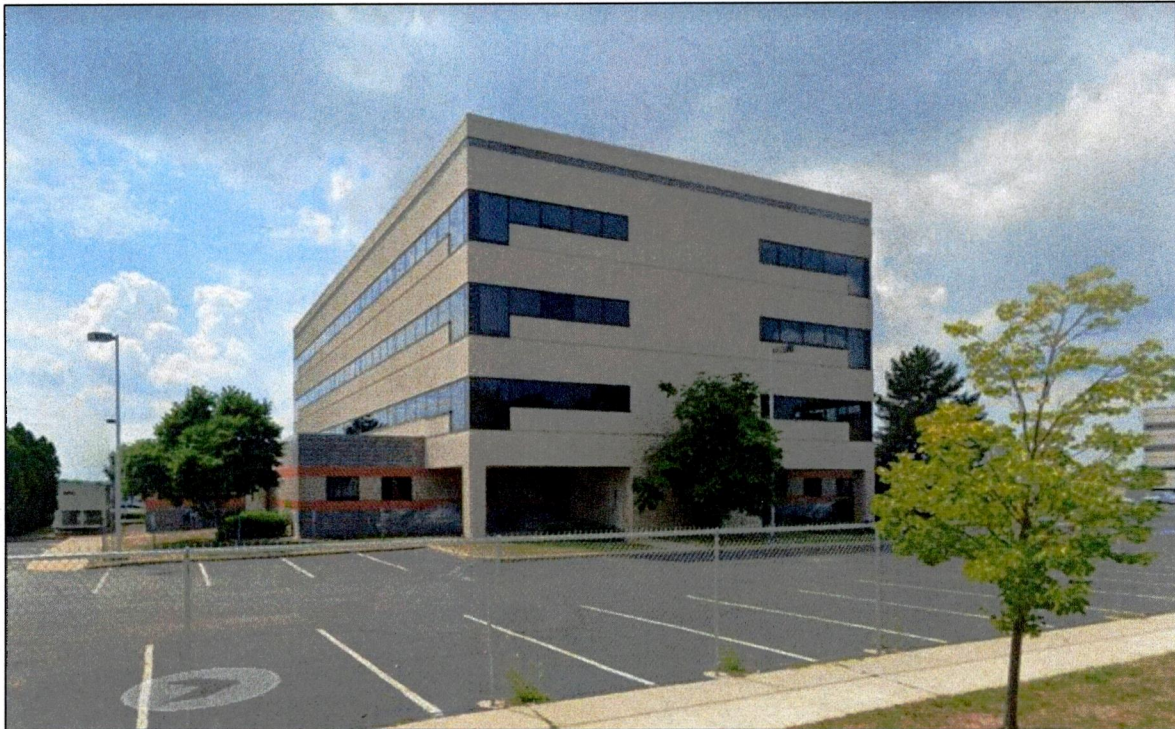
View from Miner Street looking south-southwest
