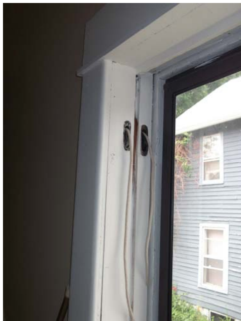
NEW SASH ROPE
