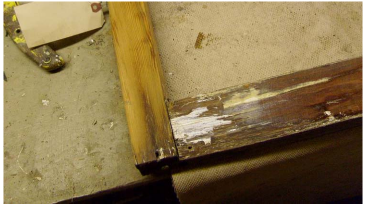
BOTTOM SASH IN PROGRESS
