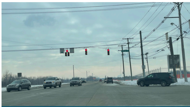
Existing Traffic Signal at Bendix Drive/Lathrop Street
