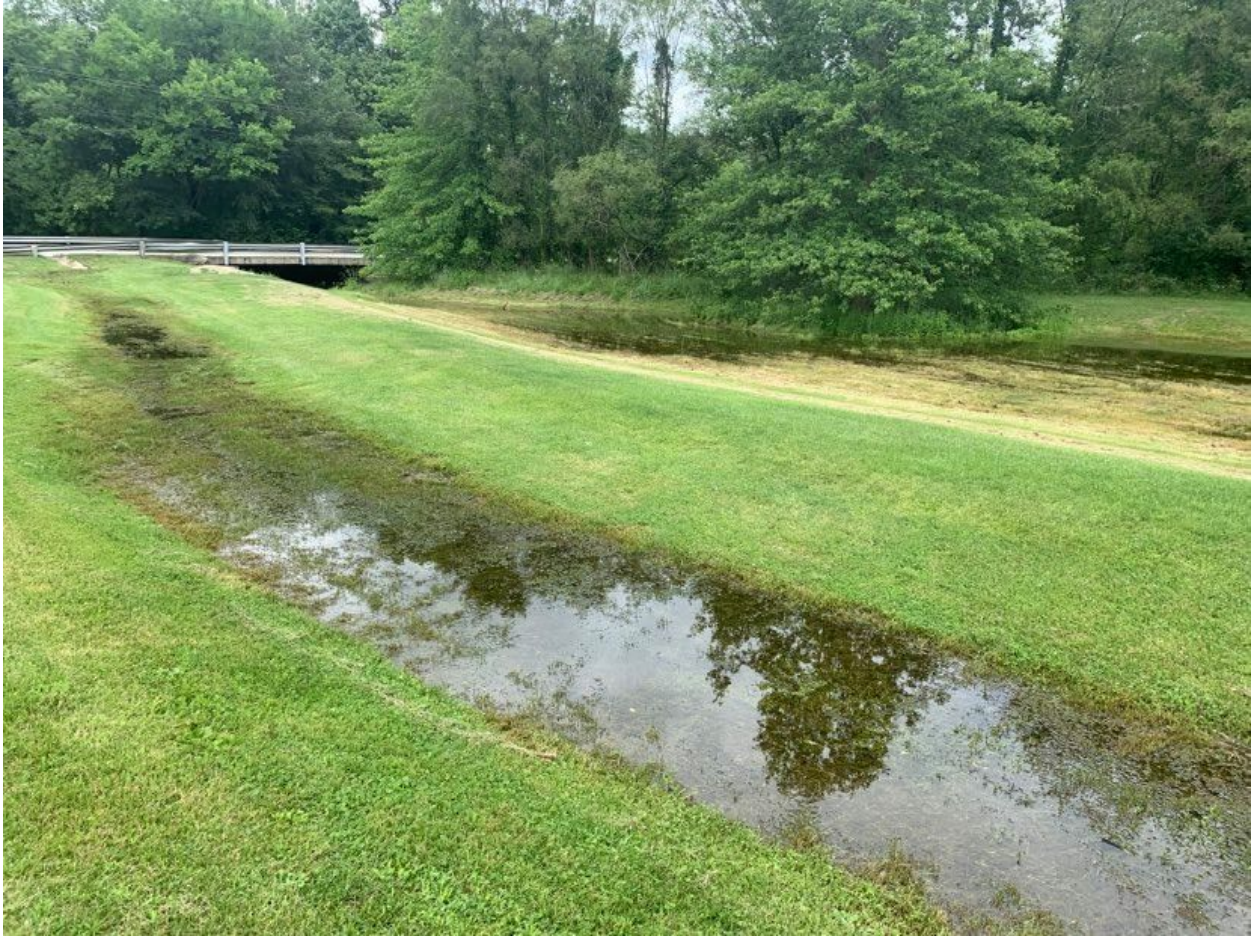
Swale at Ponader Park holding and filtering stormwater
