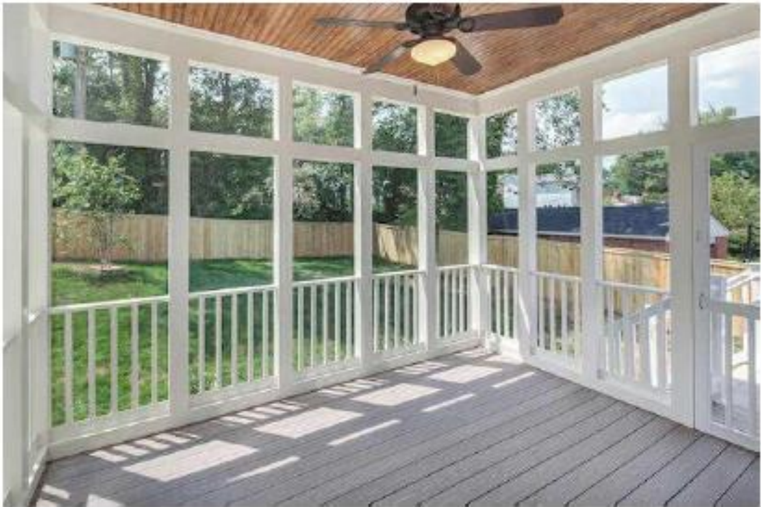
Figure 7: replacement design. Railings will be constructed from red cedar and painted white. Transoms shown in this image will not be included in the project. Decking will be sanded and stained to match ceiling.
