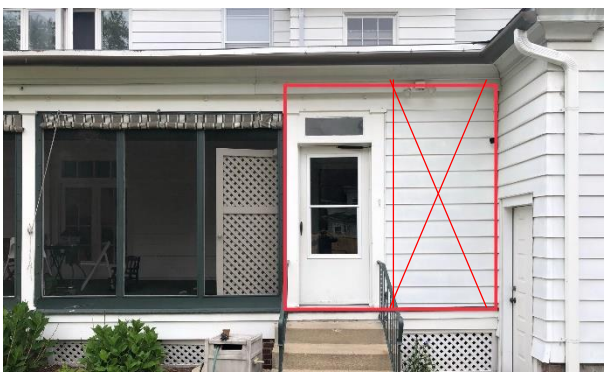
Figure 5: exterior wall added after home was originally built will be removed and replaced with railing and screen in the same style as the rest of the porch.
