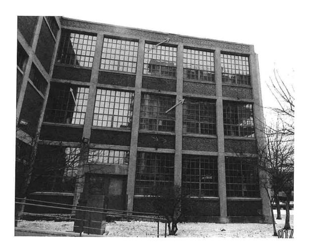
This is the chip at the top of the wall and a column with spalled concrete.
