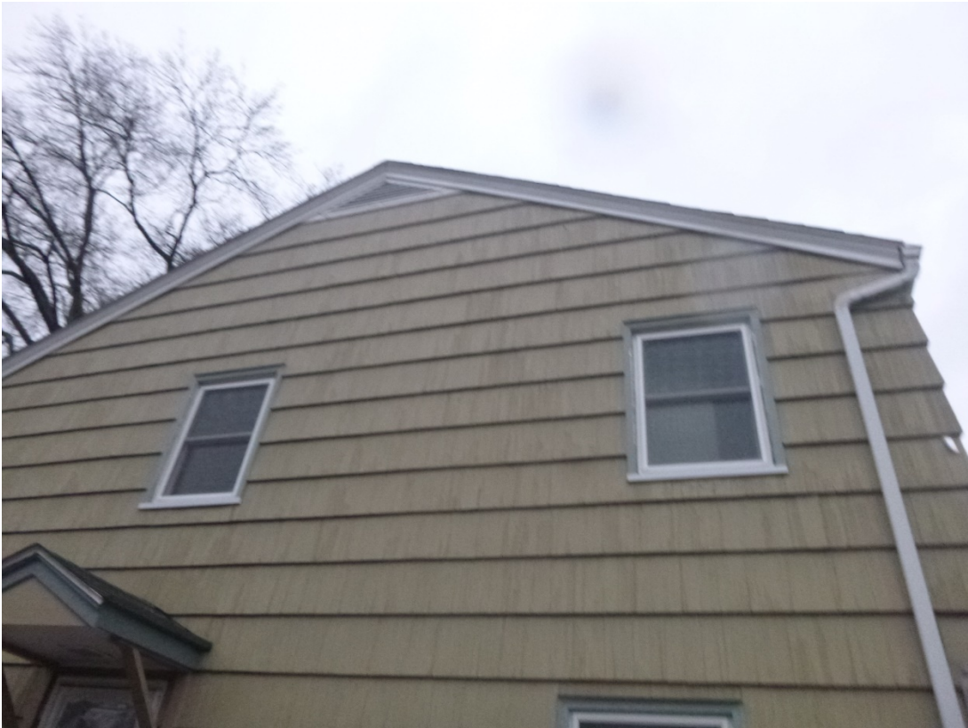
Figure 2 – East face on January 22. Upstairs windows have been replaced.
