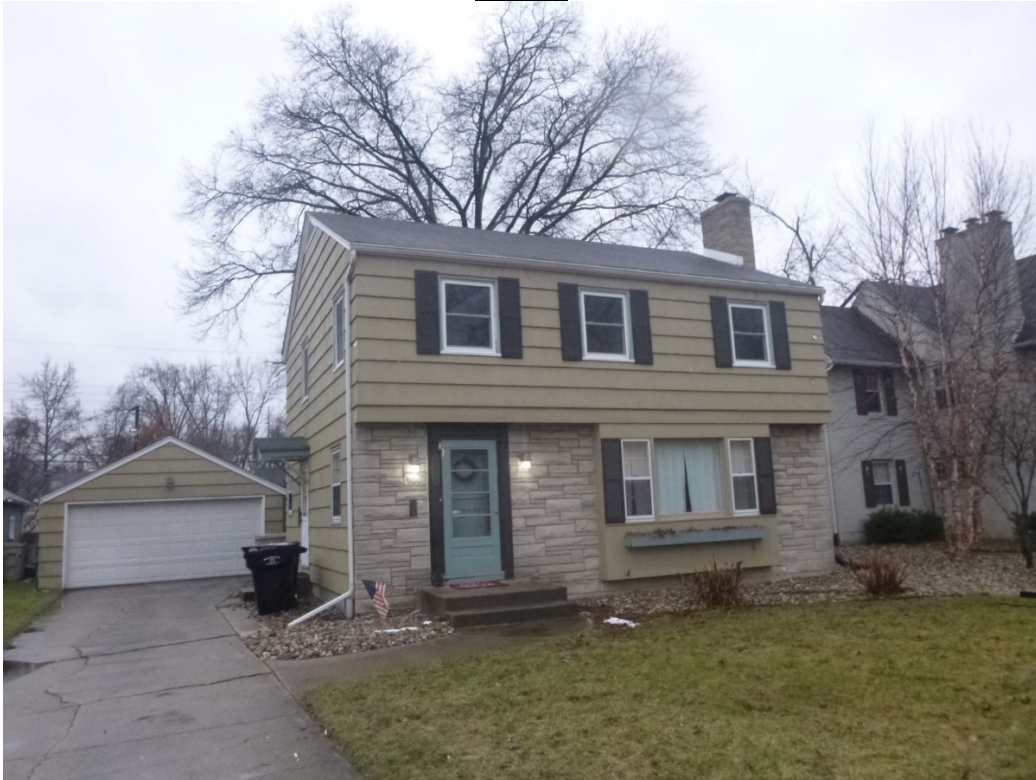
Figure 1- 1728 Wayne, taken from the Street on January 22, 2018. Second story windows have been replaced.
