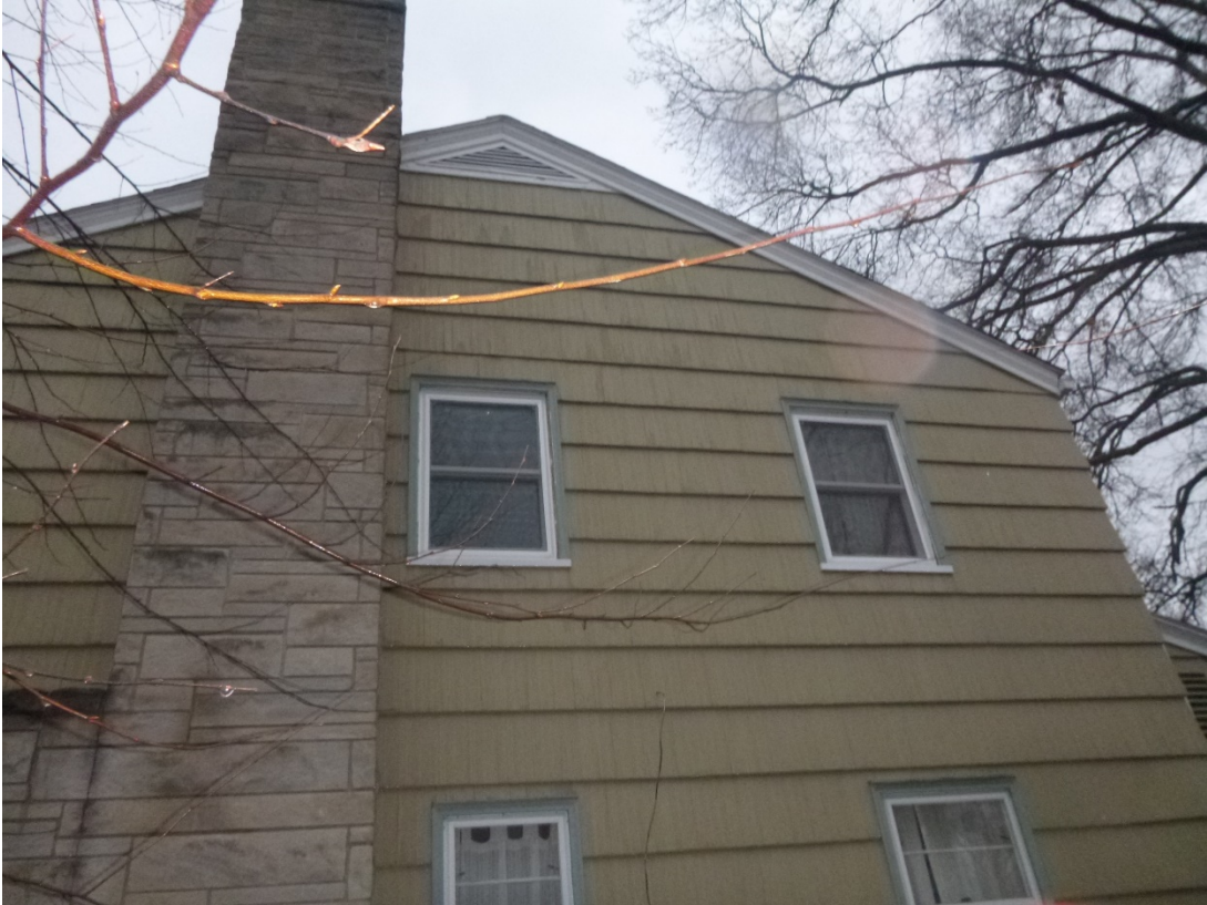
Figure 3 – West face on January 22. Upstairs windows have been replaced.
