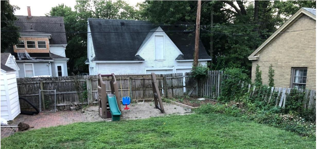
State of the fence as of August 2018. 6' privacy fence adjoining alley is missing several planks, and several posts are badly deteriorated. 4' picket fence on side of yard was overgrown with vegetation and fence posts were rotten.
