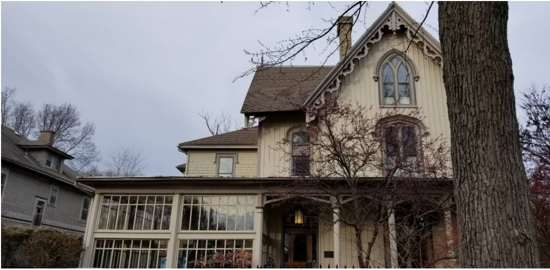
Front profile view of the house.
