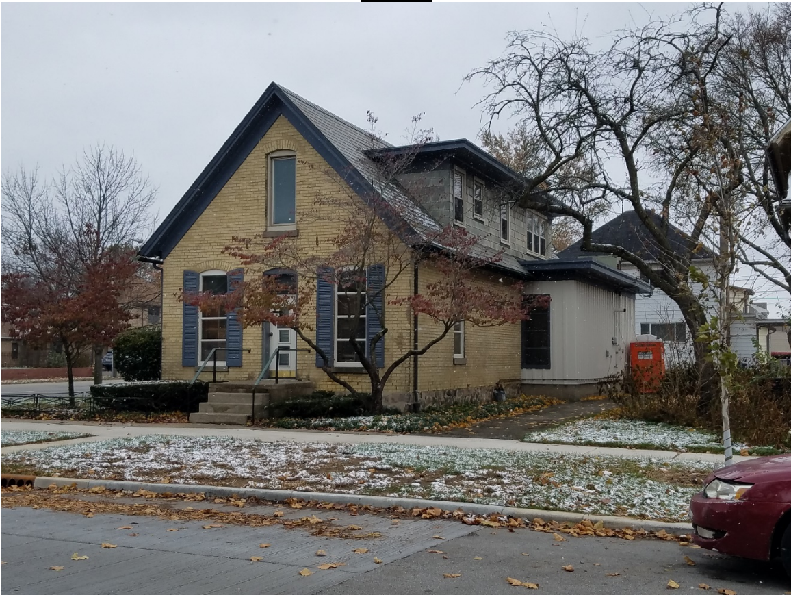
Figure 1- 1032 E Wayne from the right of way, looking south, south-east..
