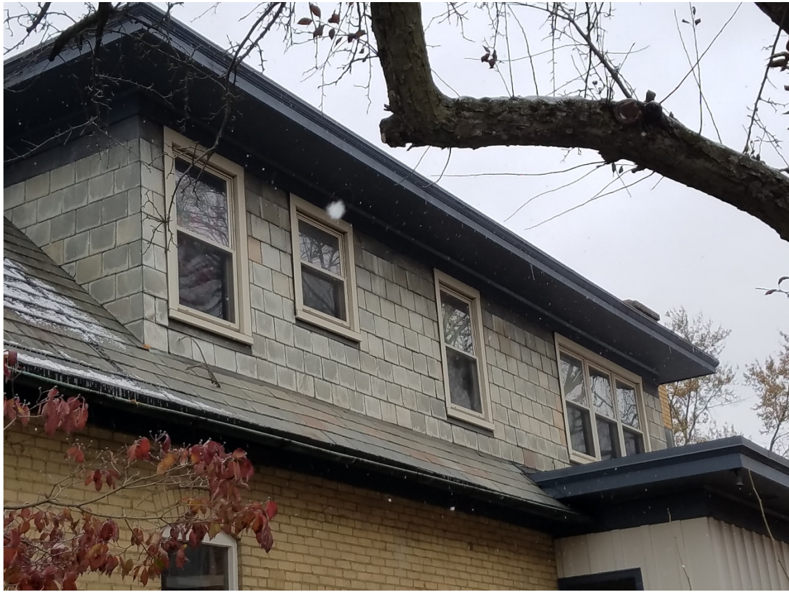
Figure 3 - West second-story dormer.
