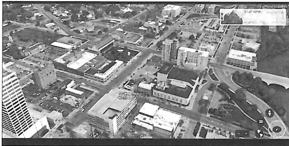
Overview of the general location of the Palais Royal building block within the downtown area
